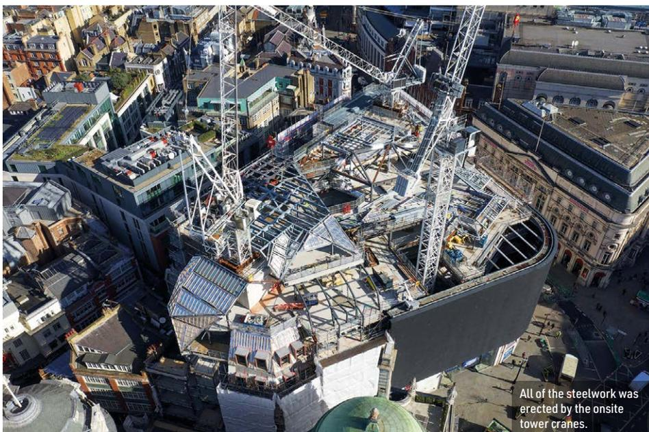
All of the steelwork was erected by the onsite tower cranes.
