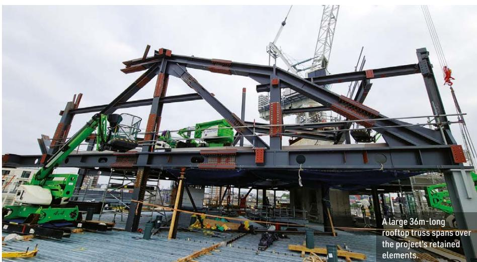
A large 36m-long rooftop truss spans over the project's retained elements.
