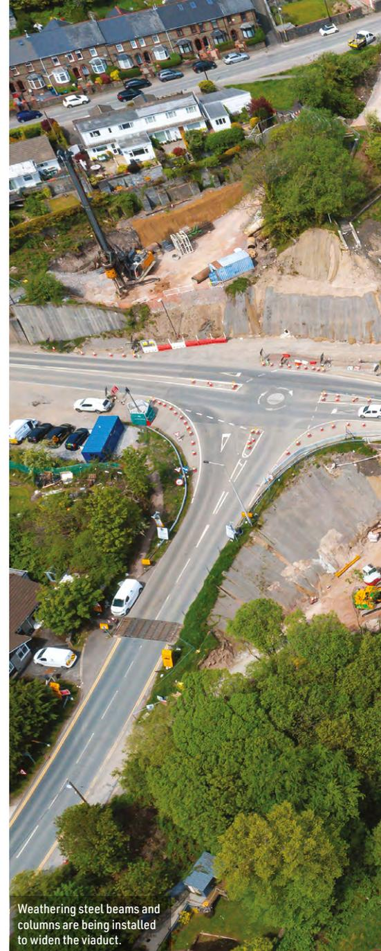
Weathering steel beams and columns are being installed to widen the viaduct.
