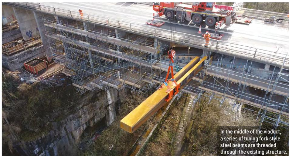
In the middle of the viaduct, a series of tuning fork style steel beams are threaded through the existing structure.
