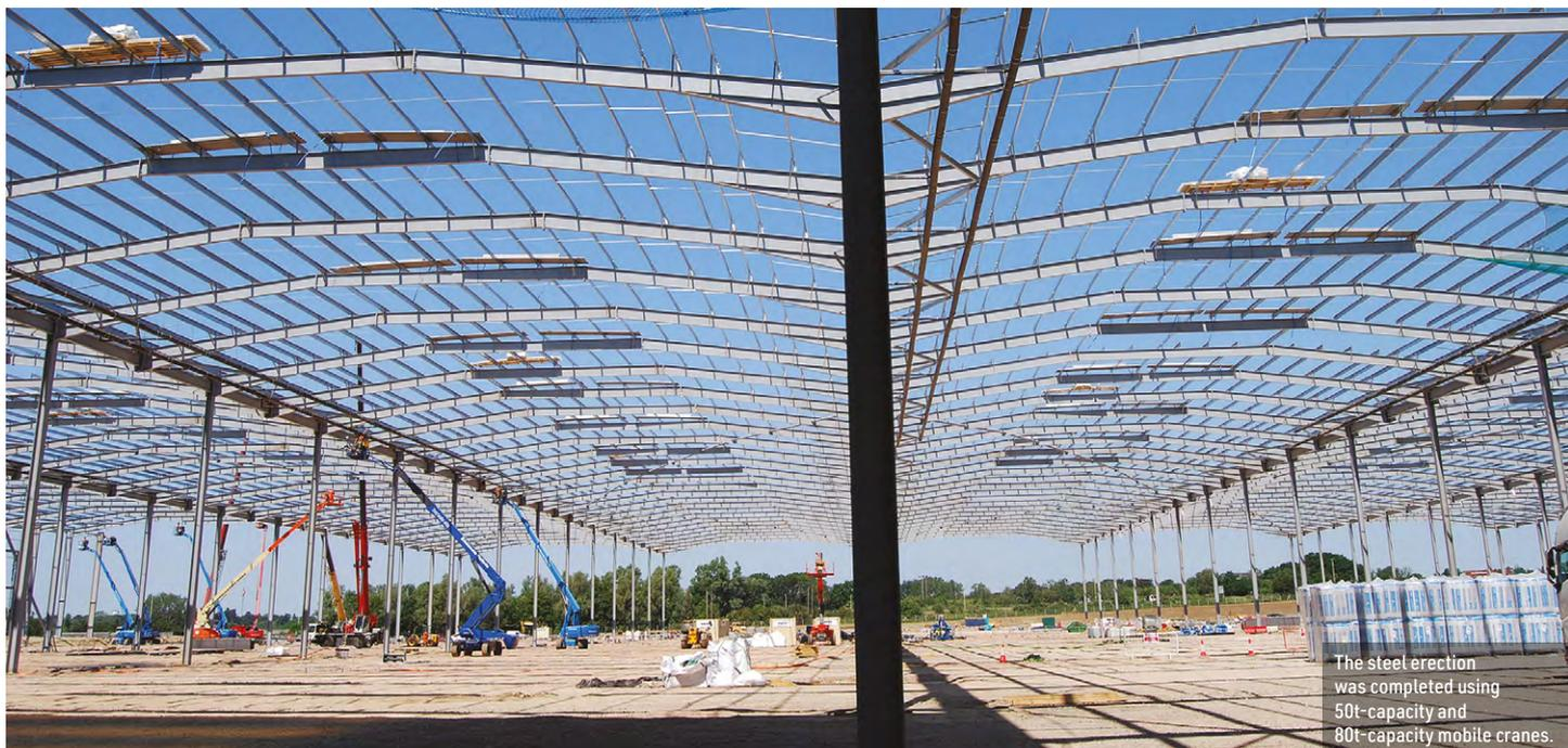
The steel erection was completed using 50t-capacity and 80t-capacity mobile cranes.
