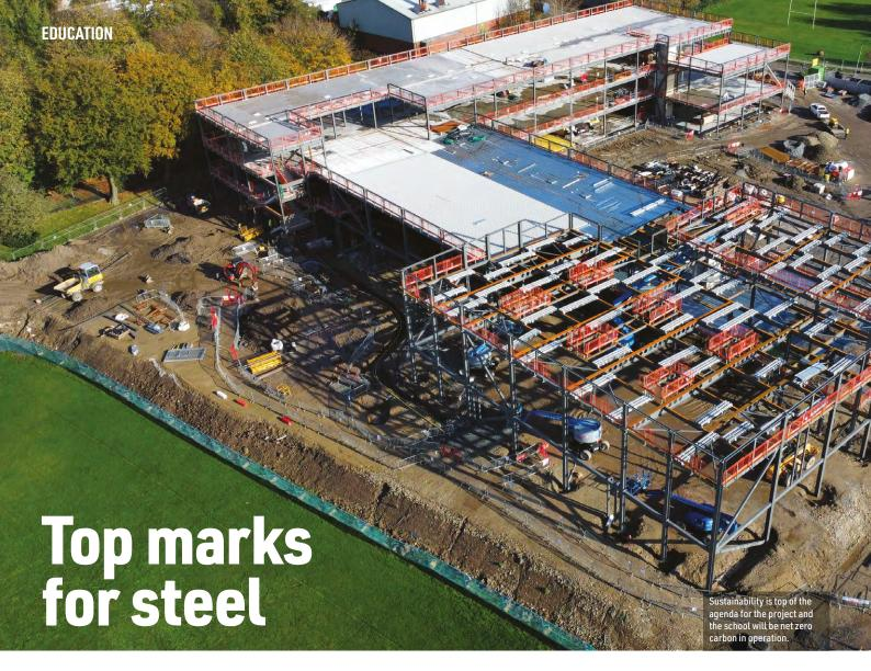
The use of structural steelwork has provided a school project in Wigan with the solution for a regular classroom column grid pattern and long spans for the sports and assembly halls.
