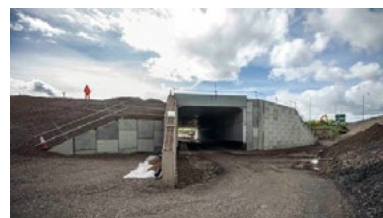
Wheatlands Road bridge in Galashiels is constructed (left)
