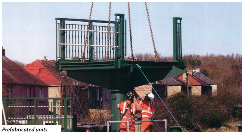
Prefabricated units are lifted into place during the construction programme
