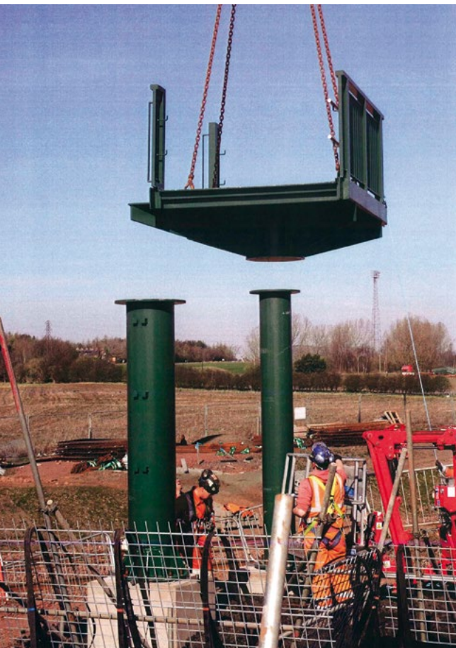
Prefabricated units are lifted into place during the construction programme
