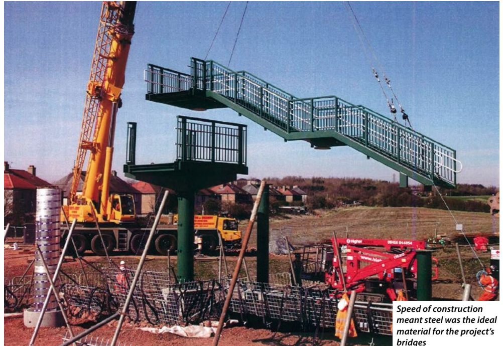
A central span is lifted into position in one piece
