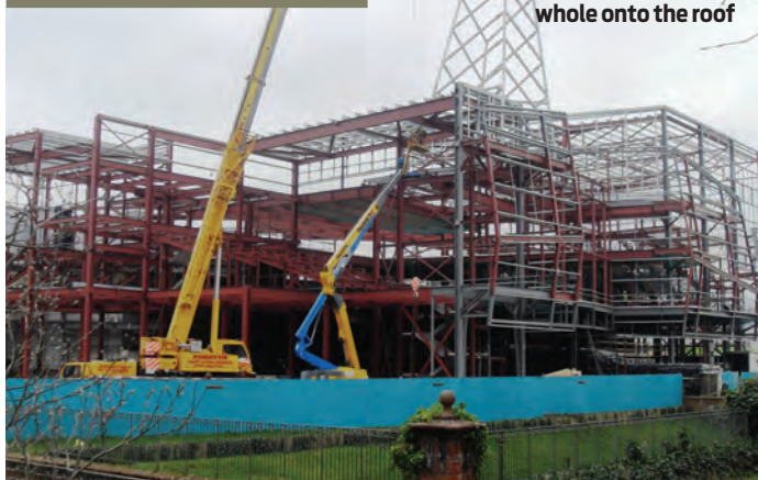
The tower was connected up at ground level before being lifted whole onto the roof
