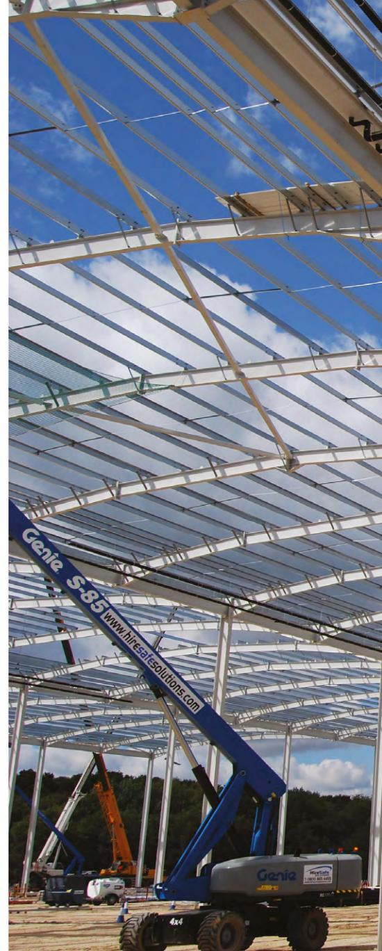
Making sure the steel frame was erected efficiently has a knock-on effect to the rest of the scheme. As once the steelwork is up, or partially up, the follow-on trades, such as cladding and roofing, are able to begin their work.
