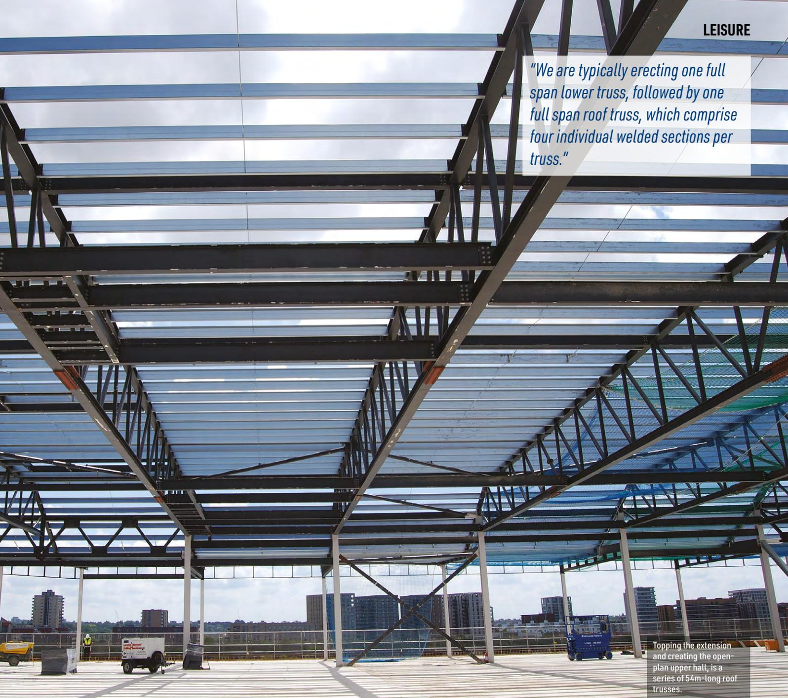
Topping the extension and creating the open-plan upper hall, is a series of 54m-long roof trusses.
