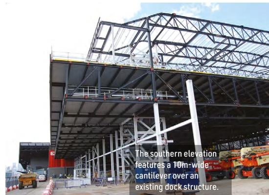
The southern elevation features a 10m-wide cantilever over an existing dock structure.
