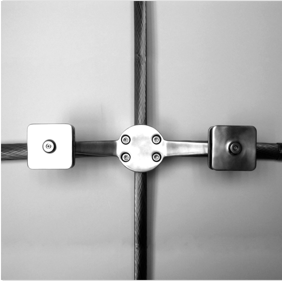
Figure 4: Close-up view of the connection of vertical and horizontal cables prior to erection (Photo: Skidmore, Owings & Merrill LLP)
