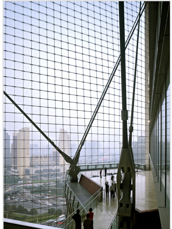
Figure 2: Main cable-net wall with primary 'v cables' (Photo: Tim Griffiths, Skidmore, Owings & Merrill LLP)
