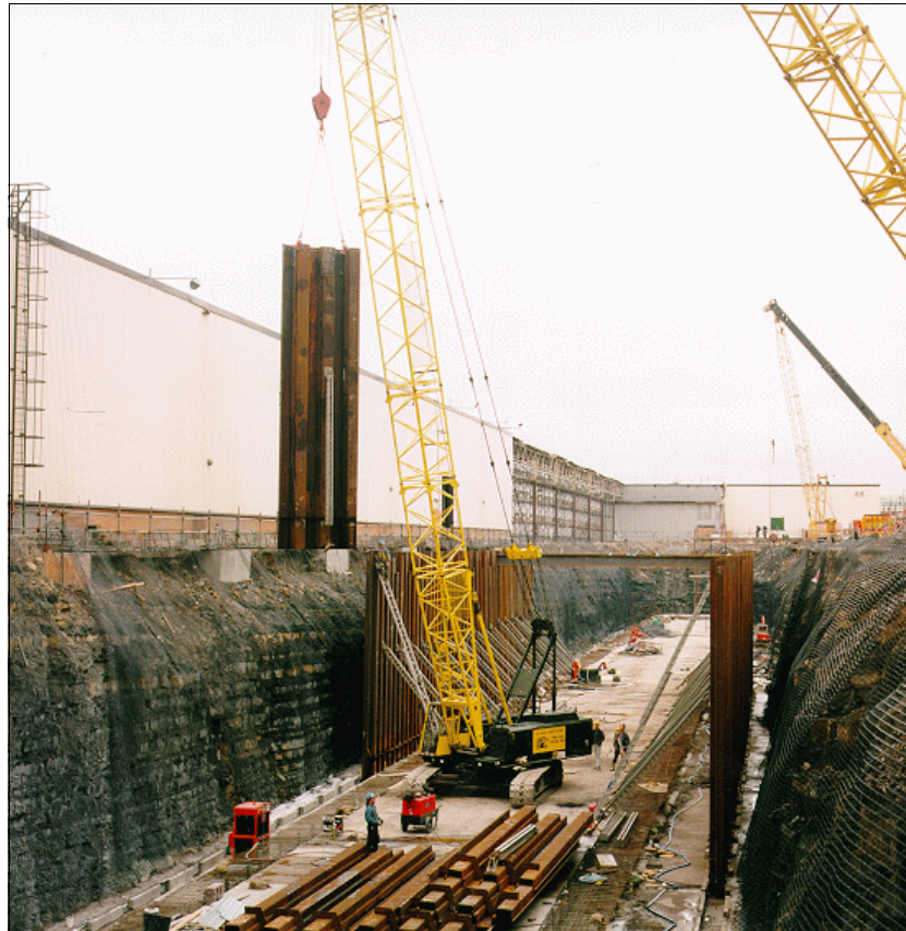
Figure 2.5 Prefabricated panels being positioned onto concrete slab
