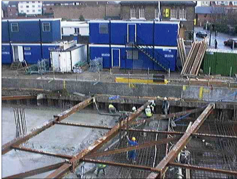
Figure 2.7 Staines underground car park
