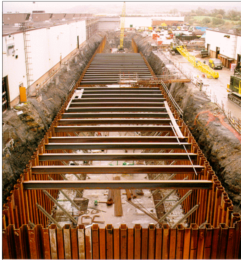
Figure 2.4 Panoramic view of the sheet pile walls and beams
