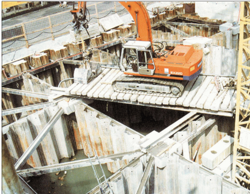
Figure 2.8 Construction of an underground garage, Rapperswil, Switzerland
