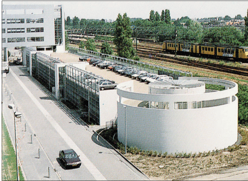
Figure 2.2 Underground car park , The Hague, Holland (TESPA)
