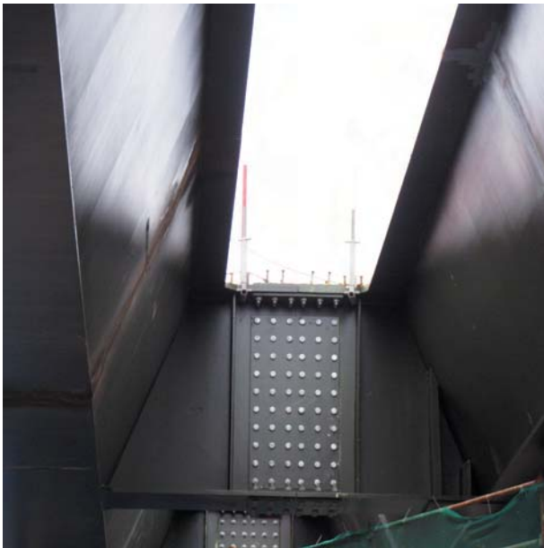
Typical Bolted Splice
