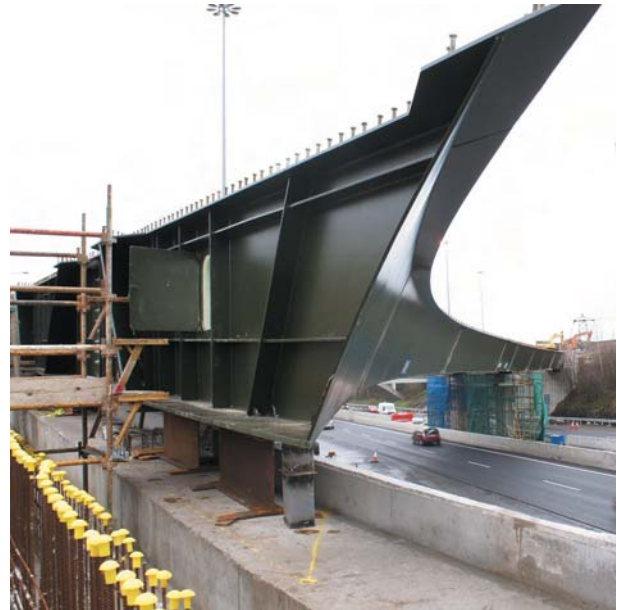
View from South West Corner
