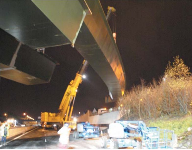
View of Lift 3 being placed
