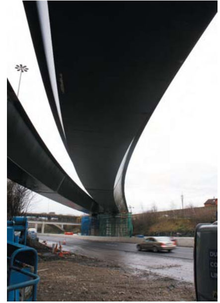
Soffit View of Lifts 3 and 4
