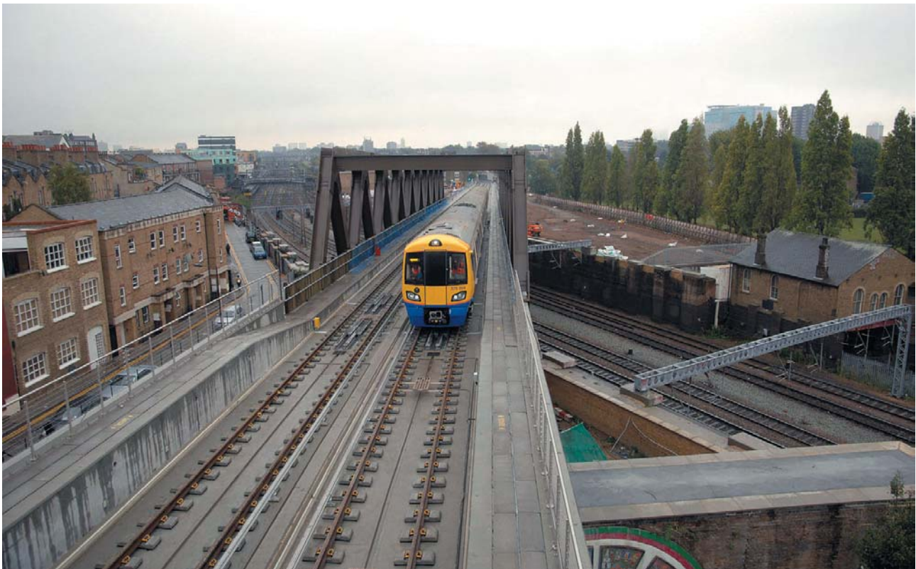
First train crossing Bridge GE19
