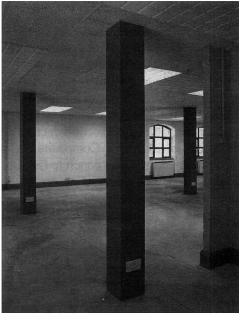
Figure 7.10 Board protection (Vicuclad, courtesy of Promat Ltd)
