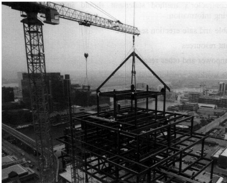
Figure 4.2 South Quay station under construction (courtesy of British Steel)
