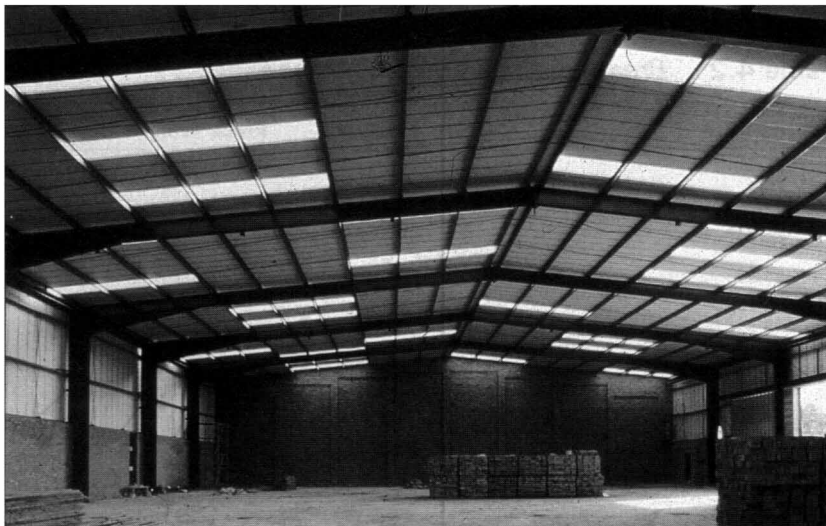
Figure 4.3 Typical portal frame
