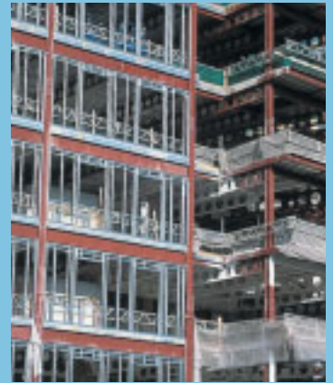
Light steel infill walls
