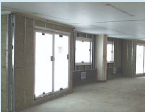
Lightweight infill walls
