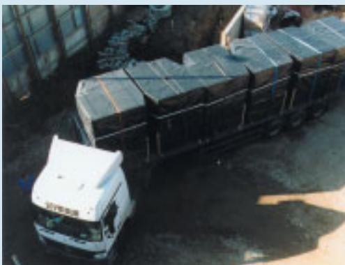
Delivery of toilet/bedroom pods
