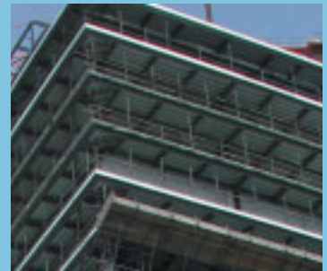
Detail of underneath of decking
