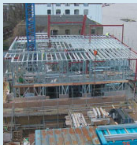
Metframe panels during construction
