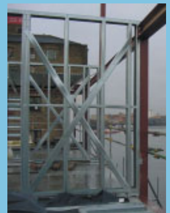
Pre-fabricated wall panels
