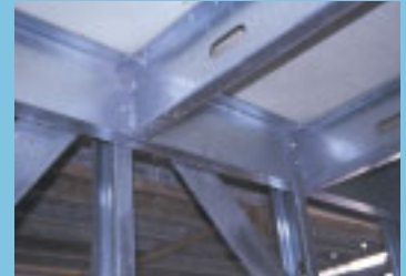
Light steel floor joists showing attachment to wall
