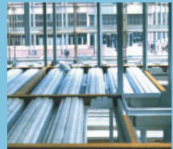
Decking supported by ASB beams
