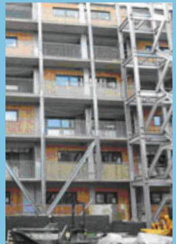
Access walkways being installed
