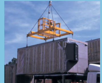
Modules being lifted into place (using man-basket)
