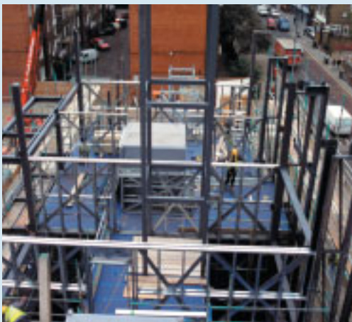
Installation of light steel frames
