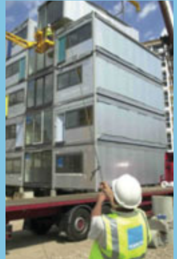
Installation of modules
