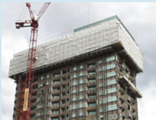
Over-roofing in progress
