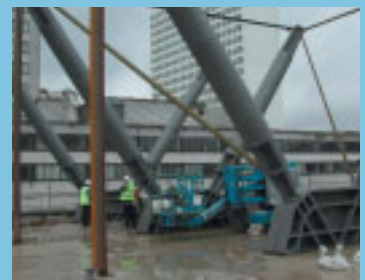
Inclined tubular legs
