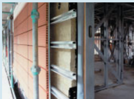
'Rain-screen' cladding during installation
