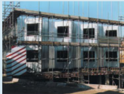
Room modules before cladding
