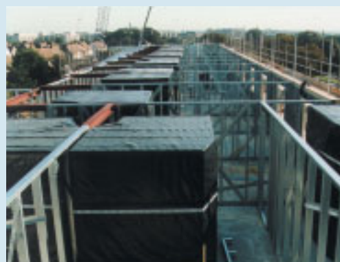
Toilet/bedroom pods in place
