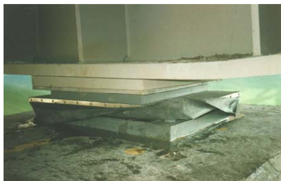
Figure 3 Guided bearing (with skirt)
