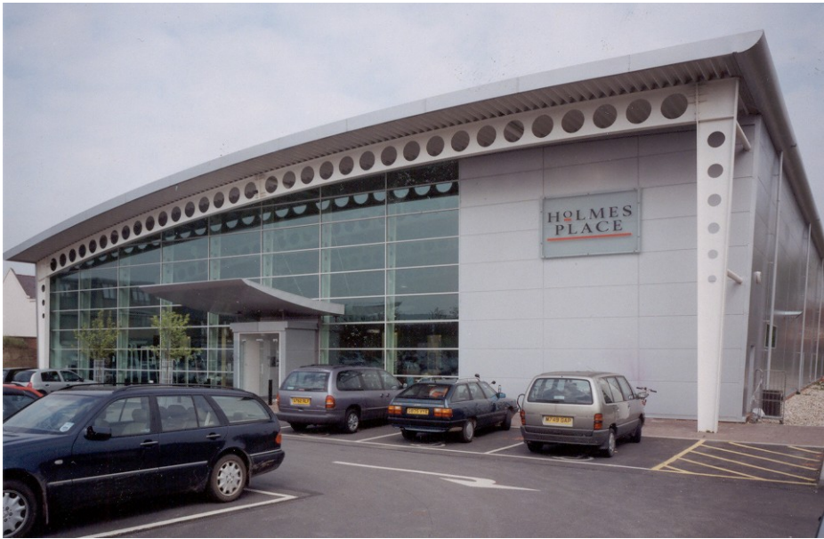
Figure 3.3 Cellular beam used in portal frames
