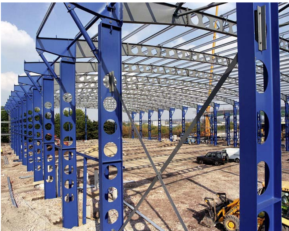
Figure 3.4 Innovative moment-resisting connections in an industrial building
