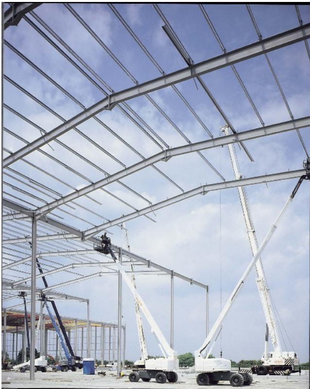
Figure 3.14 Installation process for a modern portal frame
