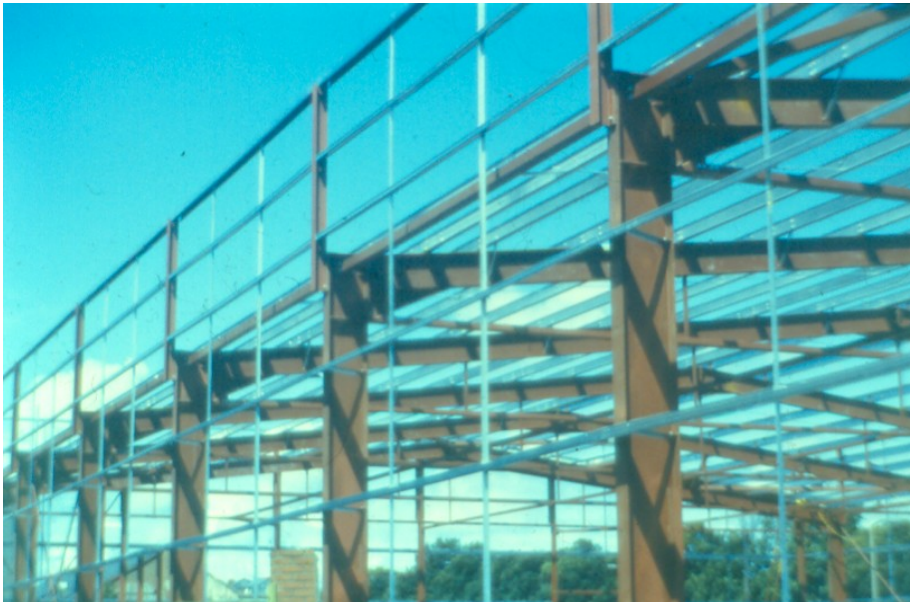
Figure 3.2 Typical portal frame and secondary components
