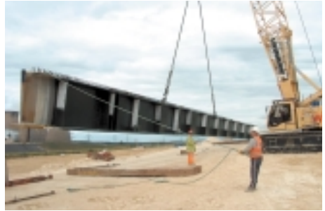
Controlling the lift
