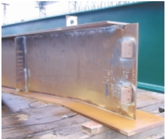
Temporary cleats in position
