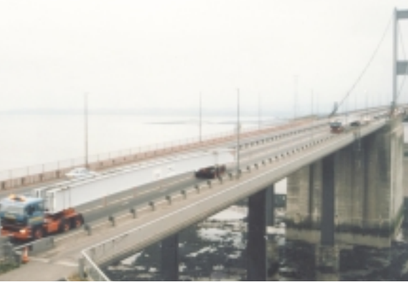
Delivery to site
