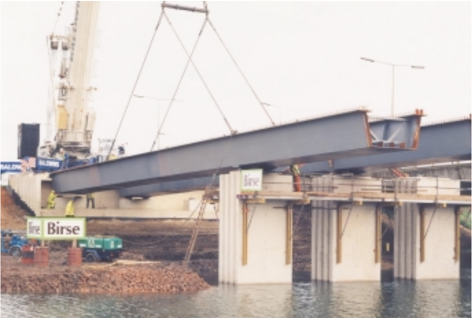
Continuous box girders
