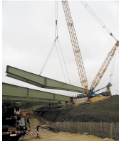
Direct erection
