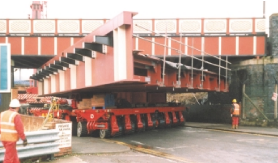
Stabilisation for movement
