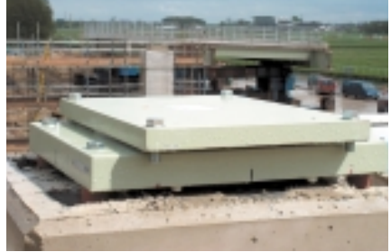
Bearings ready for the steelwork
