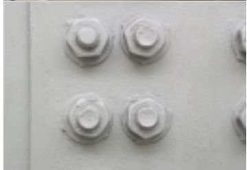
Site applied protective treatment
