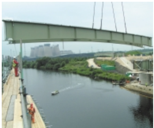
Work over water
