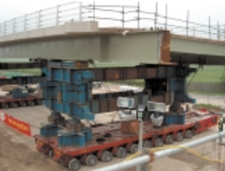
Movement of spans by transporter units
