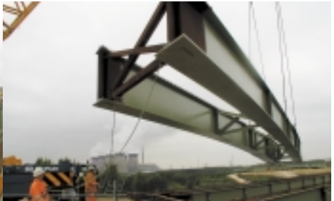
Braced pair being lifted
