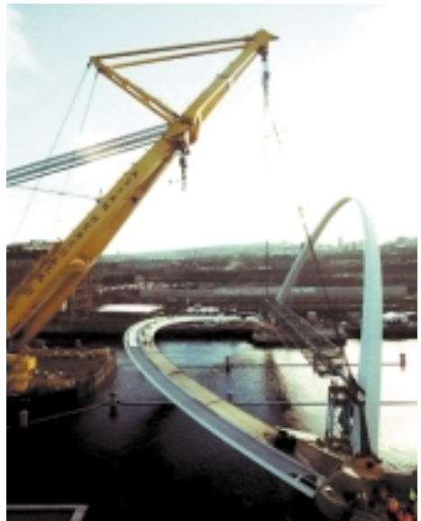
Lift by floating crane
