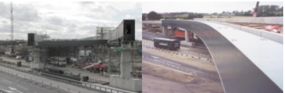
Box girders curved in plan and elevation
