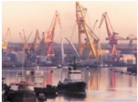
Movement of complete spans by floating crane
