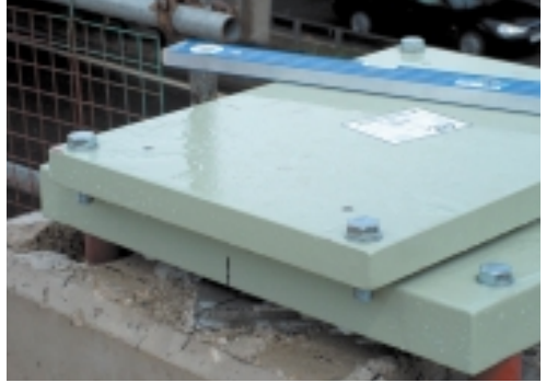
Checking the bearing for level
