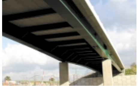
Primary beams with secondary beams
