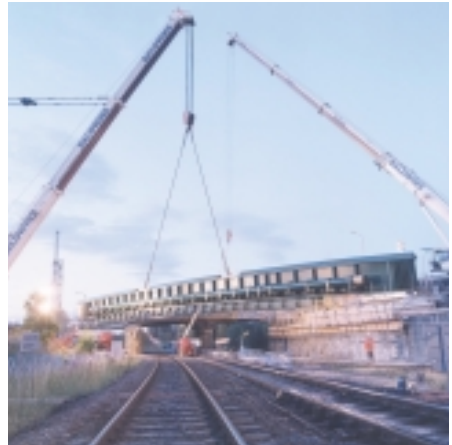
Working over a railway
