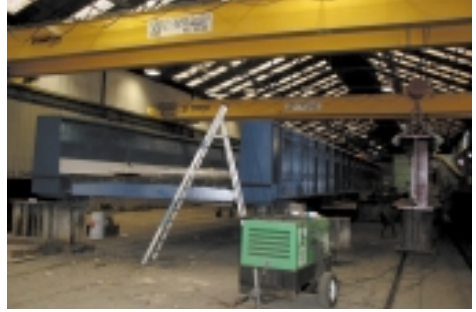
Work done in the fabrication shop
