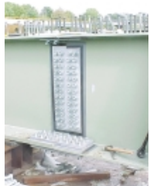
Bolted connection
