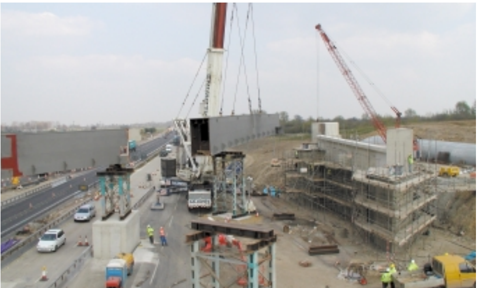
Working near a highway
