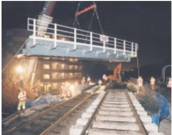
Railway underbridge being lifted in
