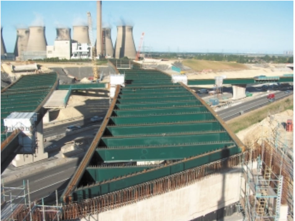
The steelwork nears completion
