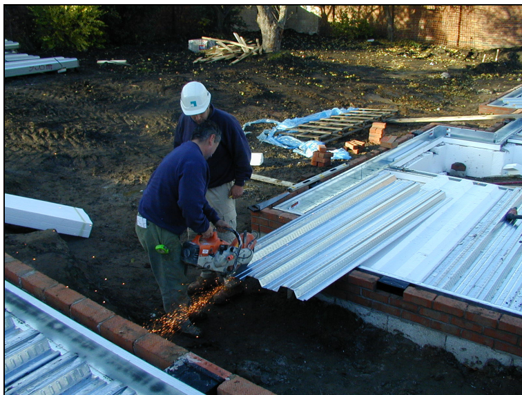
Figure 4.20 Installing a prototype composite ground floor
