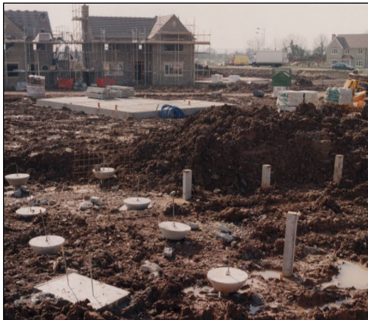
Figure 2.1 Mini-piles for houses on 'brownfield' site in flood plain
