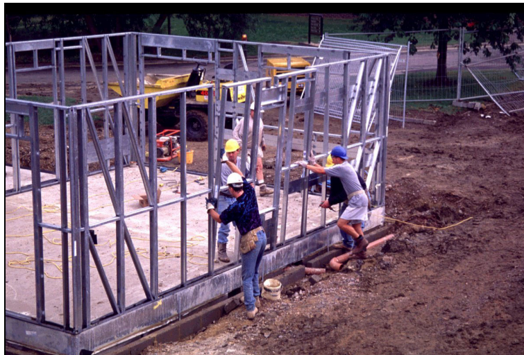
Figure 4.3 Assembling steel wall frames on composite ground floor
