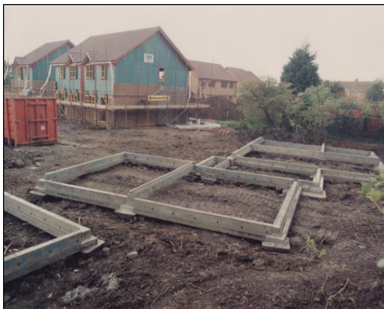
Figure 1.4 Bullivant precast groundbeam and mini-piling foundation
