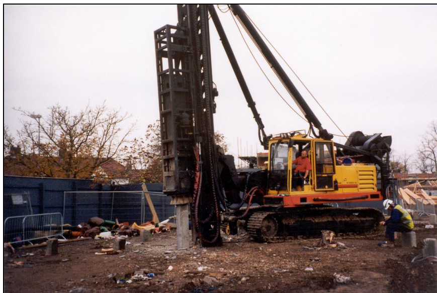
Figure 3.1 Hydraulic pile driver on precast concrete mini-piles
