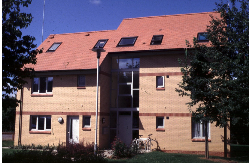
Figure 4.16 Oxford Brookes light steel framed houses
