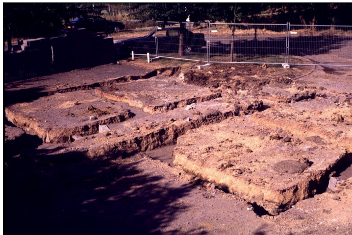
Figure 2.3 Trenchfill foundations on ‘brownfield’ site
