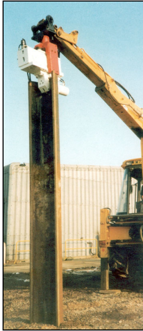
Figure 3.3 Dawson EMV pile driver mounted on excavator arm
