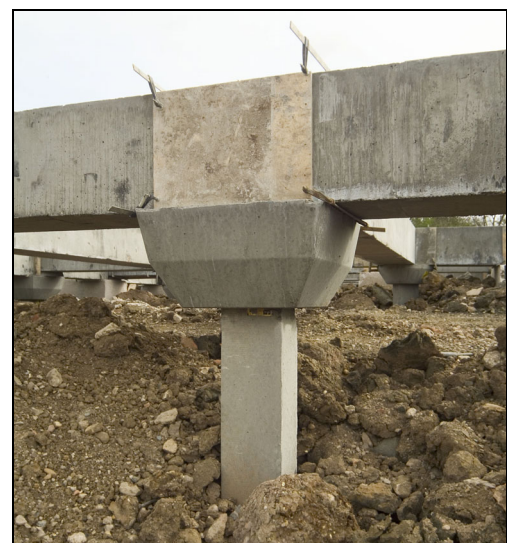
Figure 3.10 The pile, pile cap and ground beams are tied together with an in-situ concrete 'stitch'. (a) Corner joint before concreting (b) Completed joint between precast concrete beams
