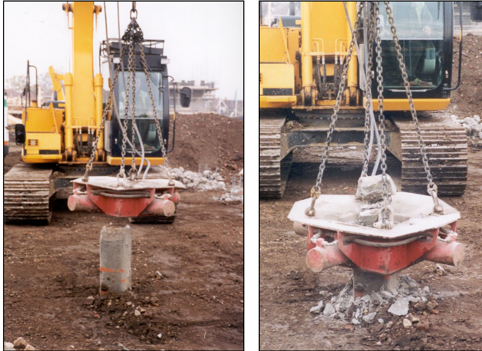
Figure 3.13 Driven precast concrete piles being cropped
