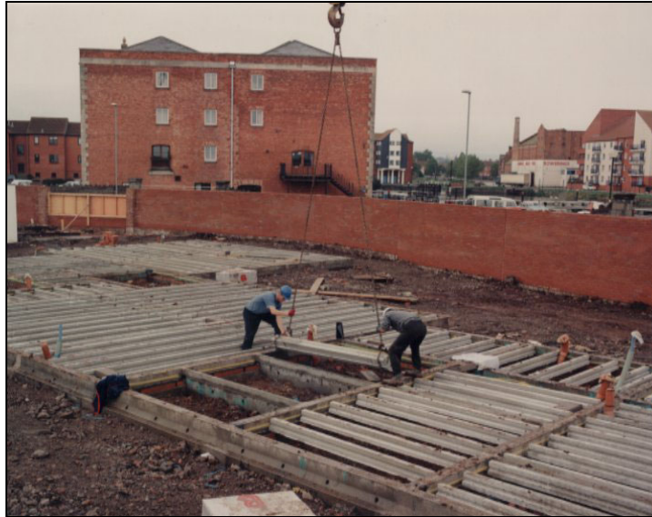
Figure 5.1 Essential use of crane for beam and block floor laying
