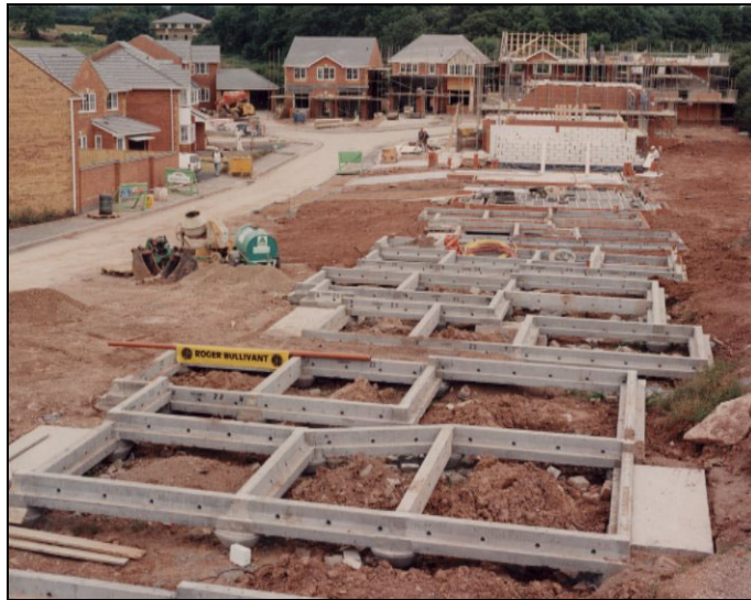
Figure 3.8 Precast ground beams awaiting precast ground floor
