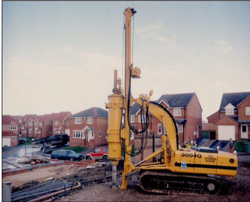
Figure 3.2 Driven precast concrete piles for housing
