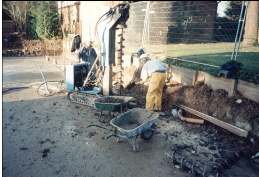
Figure 3.5 Small auger bored piling rig
