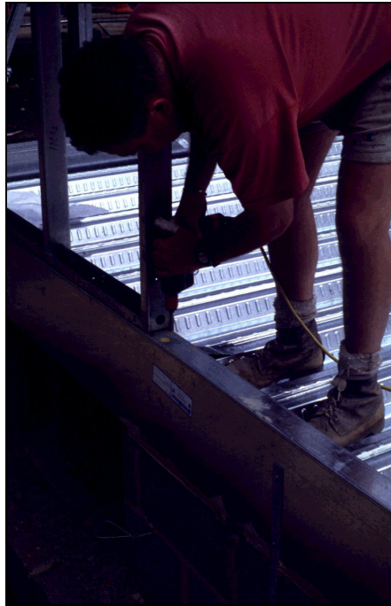
Figure 4.2 Attaching steel wall frames to the edge beam
