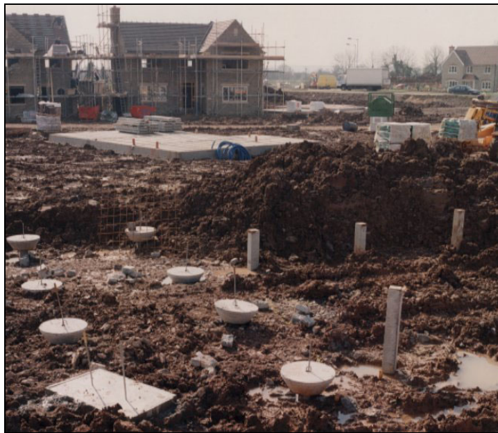
Figure 3.11 Driven precast piles before cropping
