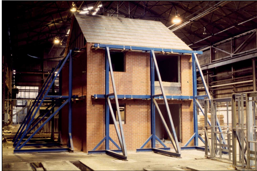
Figure 4.17 Load test on light steel frame house at Corus, Whitehead Works, Newport
