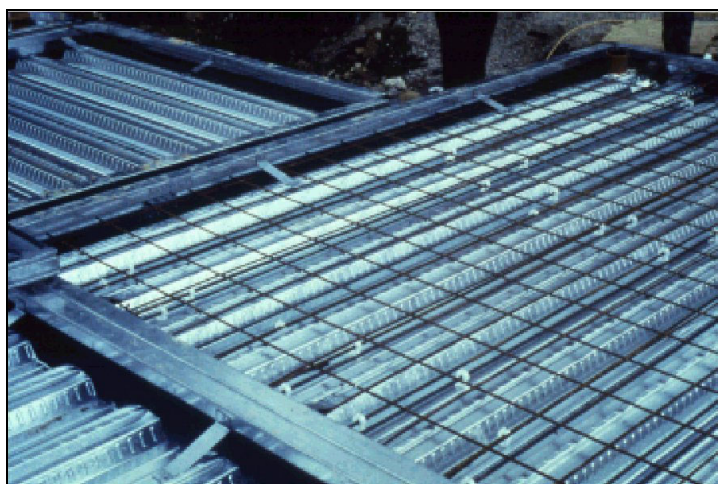
Figure 4.1 Light steel decking and edge beams before casting concrete slab
