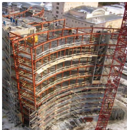
Mjärdevi Center under construction. Main framing and light steel for the exterior walls Photo courtesy of PPTH
