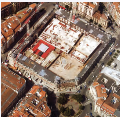
Top view of the construction site (May 2006)
