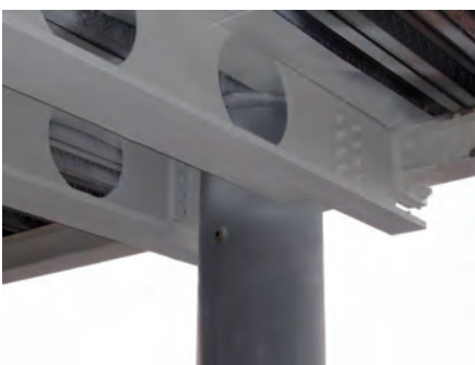
Tubular column connection
