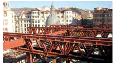
(Above) Perimeter cantilever of the atrium lattice girders
