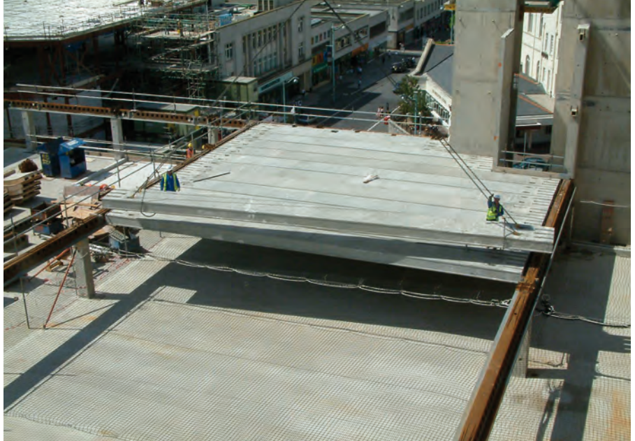
Figure 3.15 Precast concrete units placed on non-composite beams
