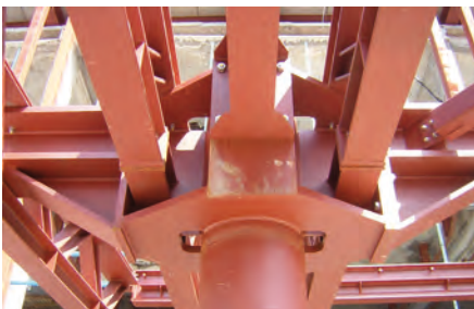
Bolted connection in a column placed in a corner between two cubes
