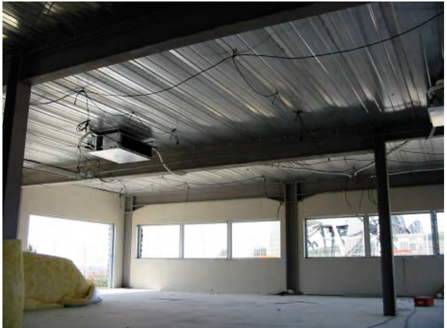
Figure 4.4 Under-side view of the finished Cofradal slab. A suspended ceiling is provided for services
