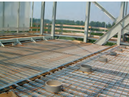
Composite slab used in the auditorium area
