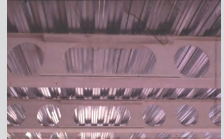
Figure 2.2 Elongated openings in beams with horizontal stiffeners
