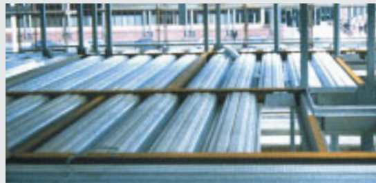
Slimdek ® eliminates the need for downstand beams
