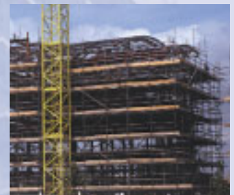
Steel frame before cladding on 4 and 6-storey development, Penarth Marina.
