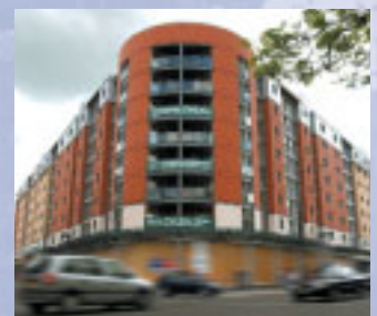
7-storey, residential student block Manchester in mixed composite and modular construction.
