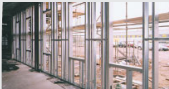
Light steel infill walls
