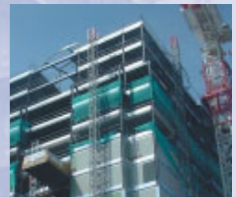
15-storey residential student block using Slimdek ® , Portsmouth.
