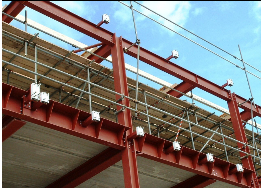
Figure 3.6 Isokorb units attached to steel frame
