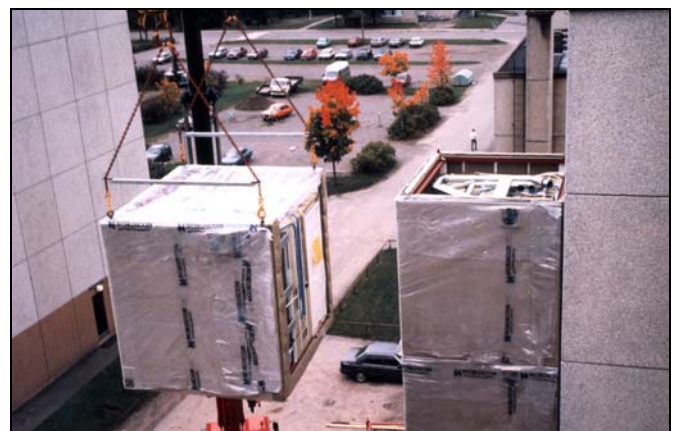
Figure 10 Open-sided bathroom modules being attached to an existing building Courtesy, Ruukki
