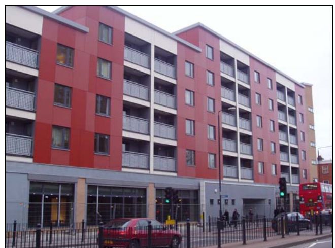
Figure 23 Mixed use of stabilising frame and modules in a residential project in Shadwell, East London Courtesy, Rollalong
