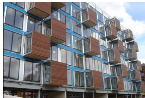
Figure 36 Balcony attachments to external structure (MoHo, Manchester) Courtesy, Shed KM Architects and Yorkon
