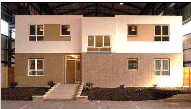
Figure 18 Demonstration building system Courtesy, Corus Living Solutions
