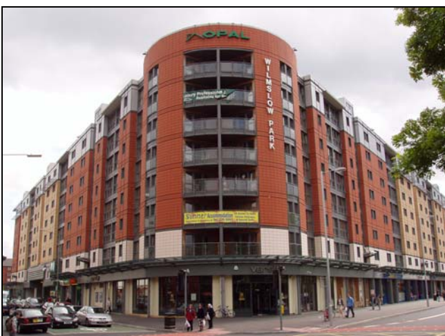
Figure 20 Typical podium structure in which seven storeys of residential units are supported on a composite frame below Courtesy, The Design Buro, Rollalong and Ayrshire Framing
