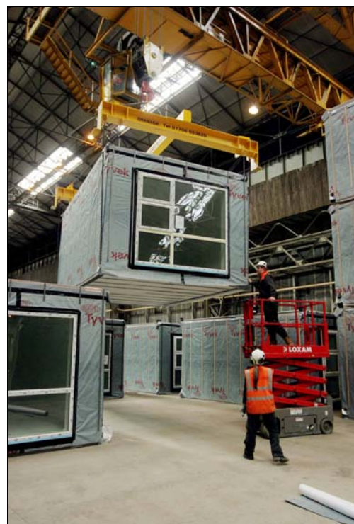
Figure 2 Module being lifted in the factory Courtesy, Corus Living Solutions
