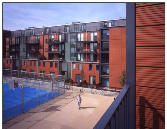
Figure 19 Mixed modular and panel building using light steel framing at Lillie Road, Fulham Courtesy, Feilden Clegg Bradley
