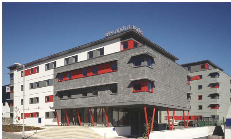
Unite Project in Plymouth; Modules supported by inclined tubular columns Courtesy, Unite Modular Solutions
