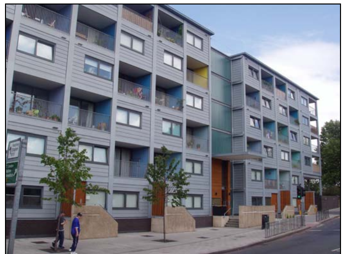
Figure 4 Raines Court, London showing integral balconies in the Yorkon modules
