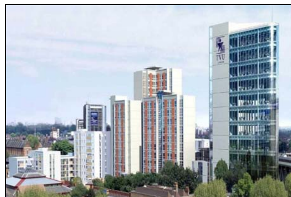
Figure 27 Concrete core used to stabilise 17 stories of modules, at Paragon, West London Courtesy, Caledonian Building Systems Ltd
