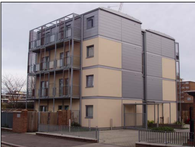
Figure 8 Completed building (above), Barling Court, Stockwell, London
