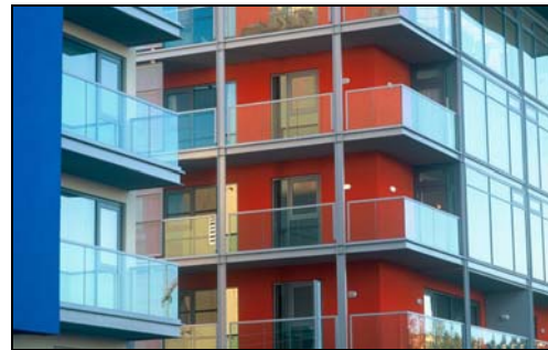
Figure 35 Self-standing balcony Courtesy, Feilden Clegg Bradley
