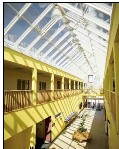
Figure 37 Atrium created between modules Courtesy, Yorkon
