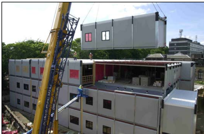
Figure 15 Modular hospital building during installation of open-sided modules Courtesy, Yorkon
