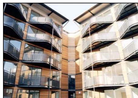
Courtyard view at Murray Grove, London showing pre-fabricated balconies Courtesy, Cartwright Pickard Architects and Yorkon
