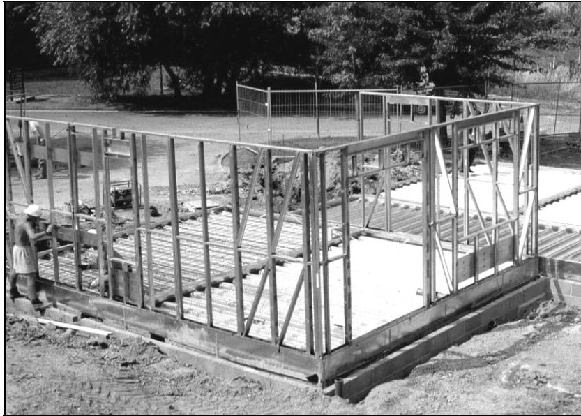
Figure 1.1 Installation of ground floor walls in light steel framing for housing
