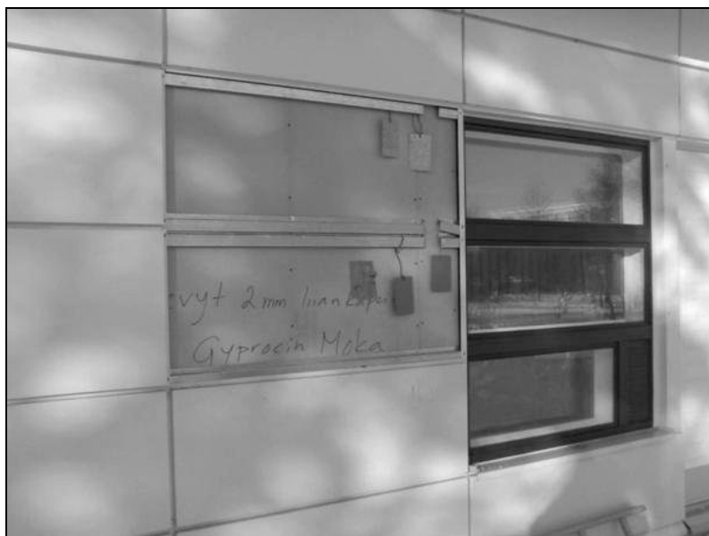
Figure 3.16 Coupons in cold cavity behind over-cladding system in Hameenlinna, Finland
