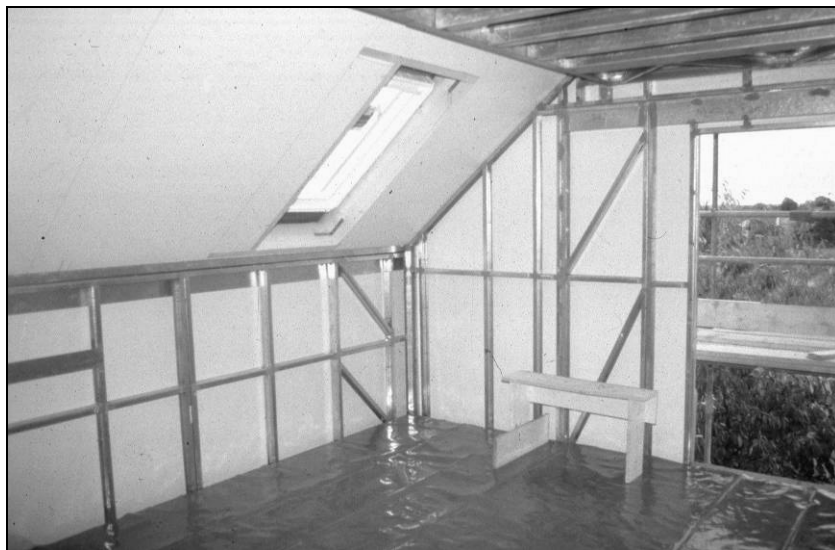
Figure 3.5 Open-roof system in the Oxford Brookes House
