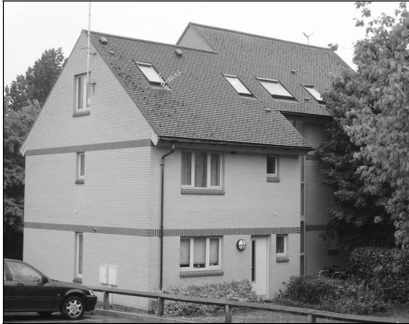
Figure 3.4 Oxford Brookes Demonstration Building
