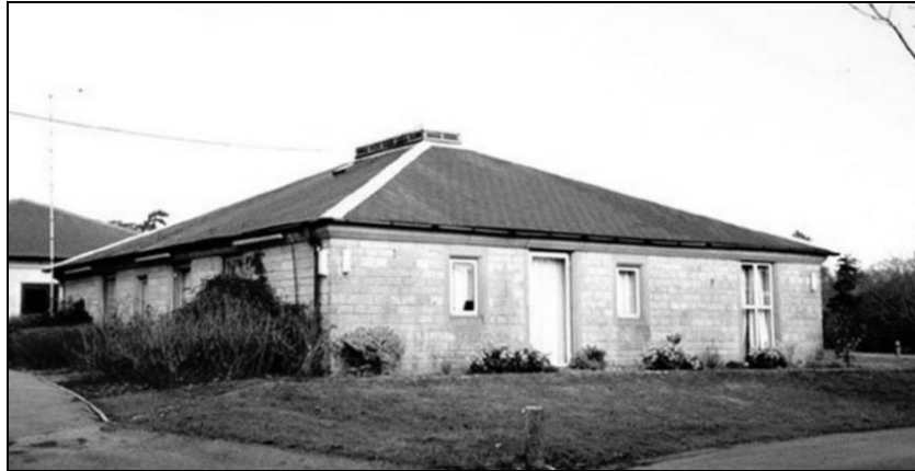
Figure 3.2 Light steel framed building for disabled persons at Ullenwood
