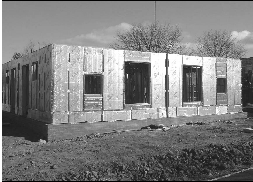
Figure 1.2 'Warm frame' construction showing external insulation
