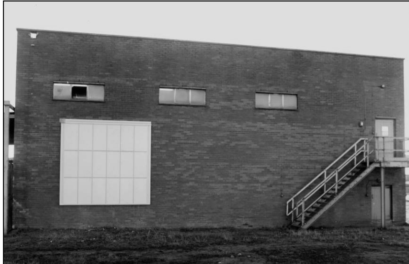
Figure 3.13 Over-cladding panel on industrial site in Port Talbot
