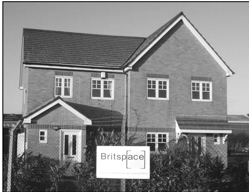
Figure 3.14 Light steel modular houses in Yorkshire
