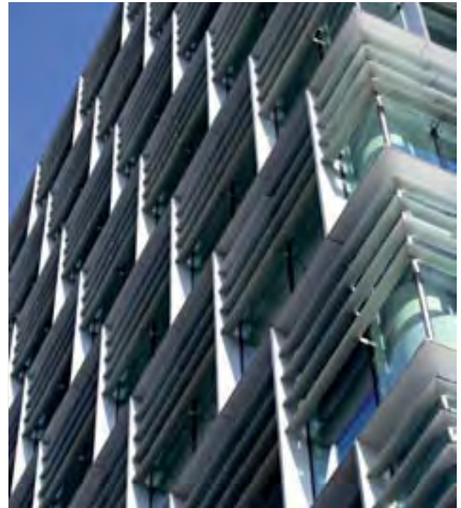
ONE KINGDOM STREET, LONDON – FAÇADE
