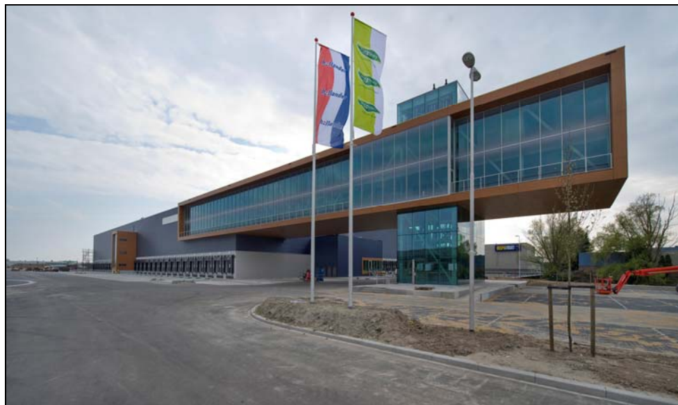
Figure 2.7 Distribution centre, Barendrecht, NL showing the braced cantilever office structure
