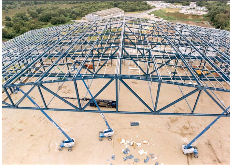
Figure 4.3 Truss fabricated from rolled sections
