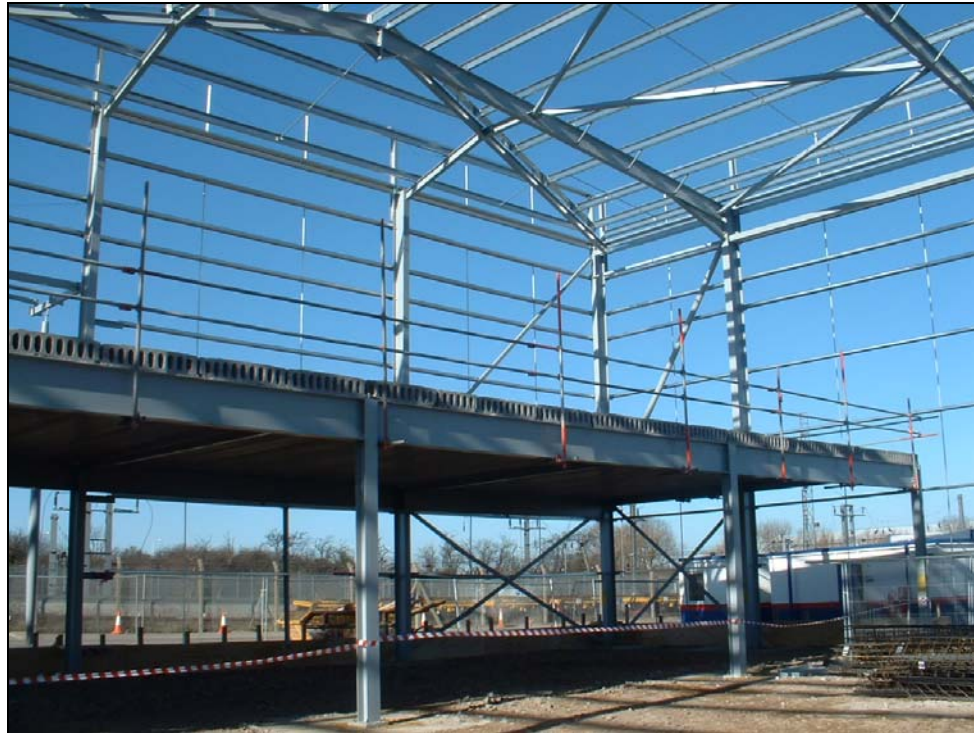
Figure 3.17 Portal frame with intermediate floor
