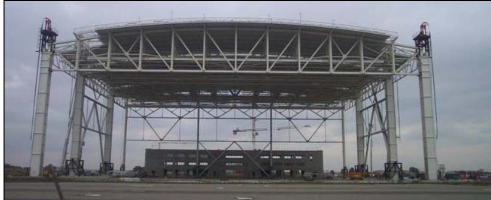
Figure 2.5 View of Airbus Industrie hanger during construction
