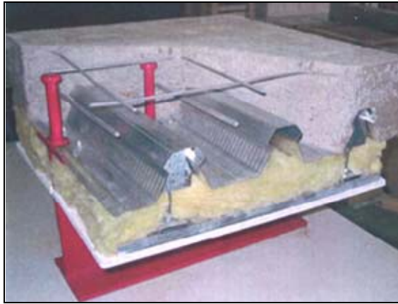
Figure 4.19 Composite slab with thermal insulation
