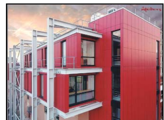
Industrial workshops for public transportation company - Paris
