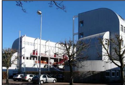
Steel cladding – Montargis (France)
