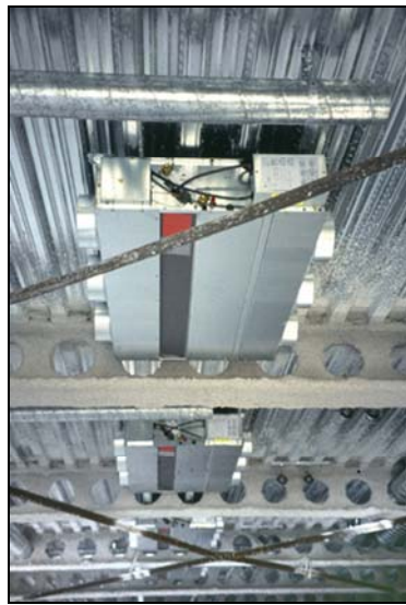
Figure 6.10 Cellular beams and service integration
