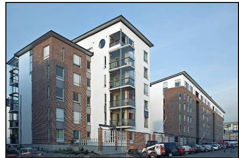
Render on load-bearing walls – Helsinki (Finland)
