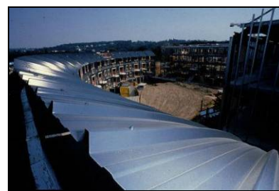
Pitched roof on site
