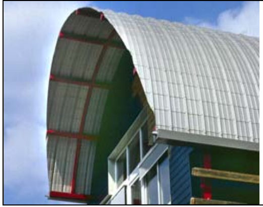
Figure 5.15 Curved roof with galvanized steel sheet
