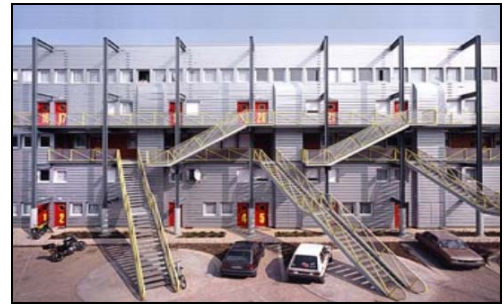
Steel cladding – Montargis (France)
