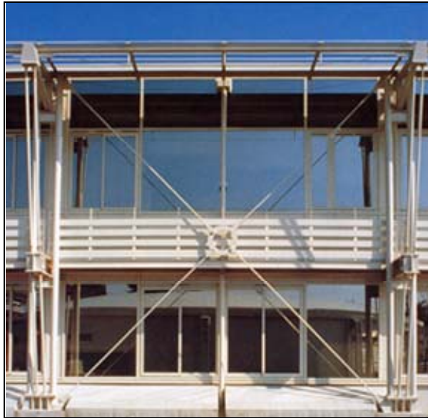
Figure 4.12 External cross-bracing in a multi-storey building
