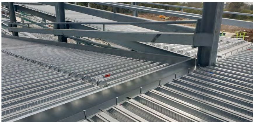
Installed Deck Picture
