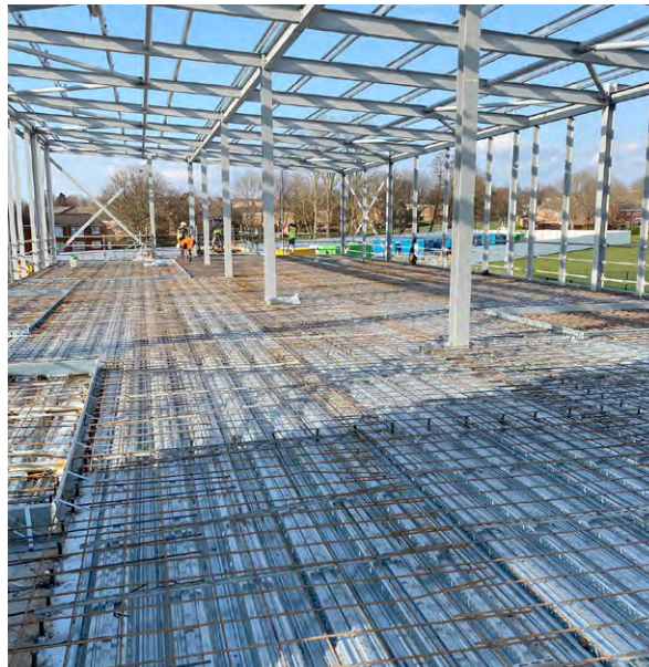
Figure 6.3 Decking and fabric reinforcement – ready for casting the concrete
