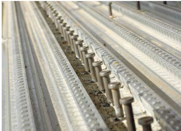
Figure 5.8 A run of stud shear connectors
