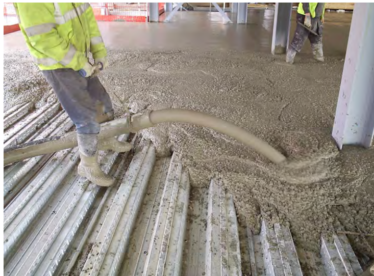
Figure 6.4 Pumping of fibre-reinforced concrete
