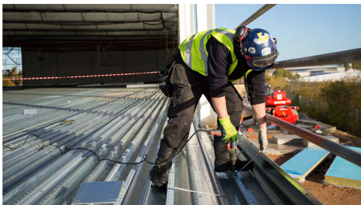
Figure 4.16 Setting out of edge trim
