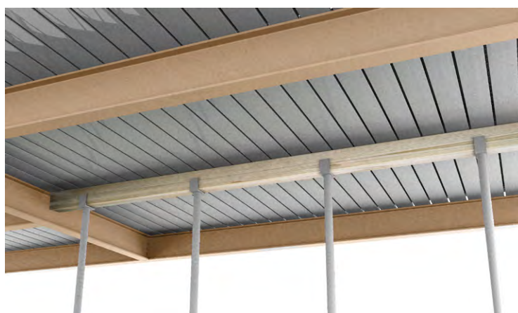
Figure 4.18 Temporary support using 'Acrow' props
