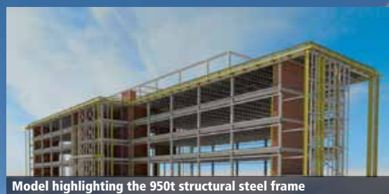
Model highlighting the 950t structural steel frame
