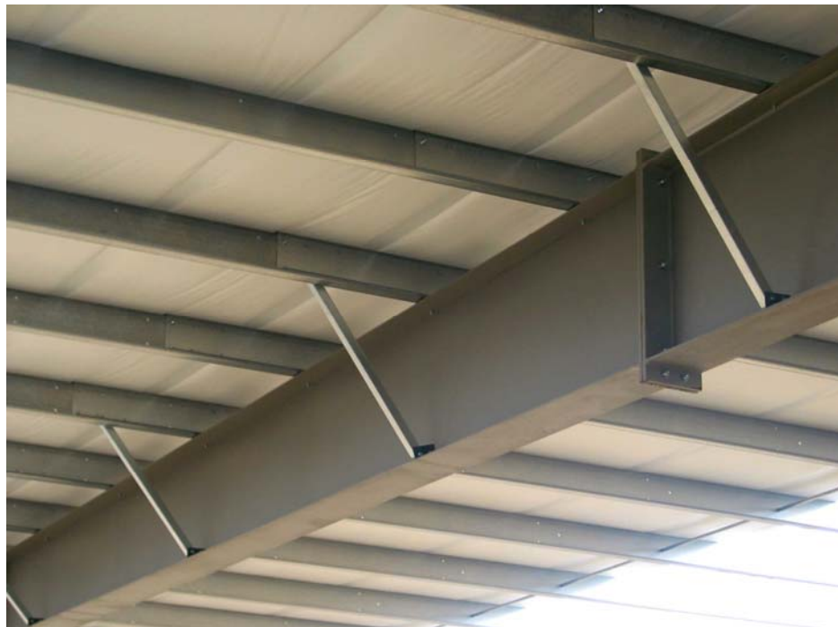
Figure 3.6 Stabilizing the bottom flange of a roof beam
