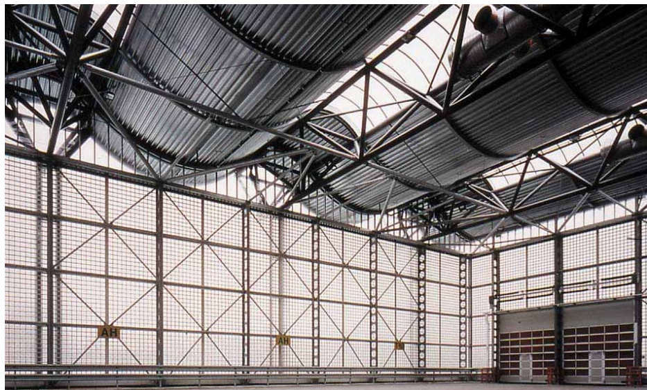
Figure 3.19 Three-dimensional trusses supporting a roof
