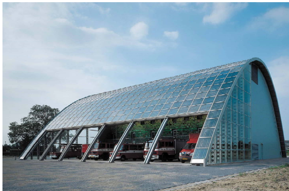
Figure 3.23 Fire brigade station
