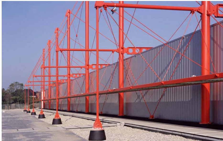
Figure 3.20 Cable stayed roof beams of a storage facility
