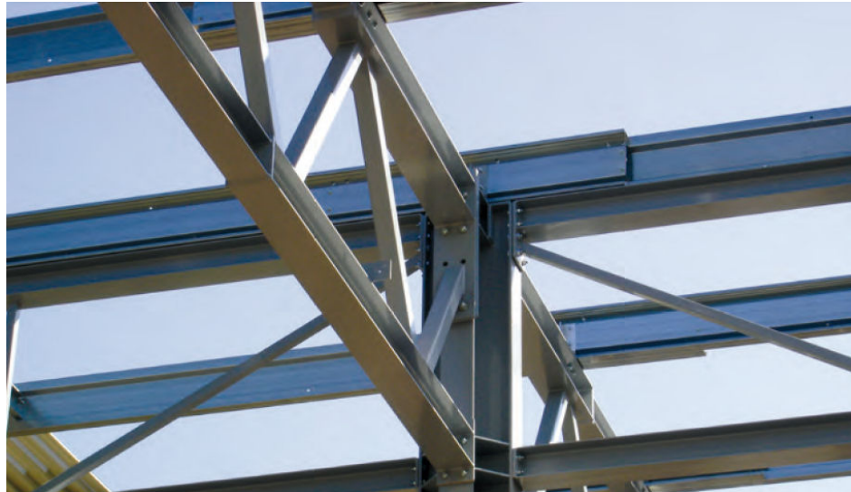
Figure 3.25 Truss-column connection in a rigid framed structure
