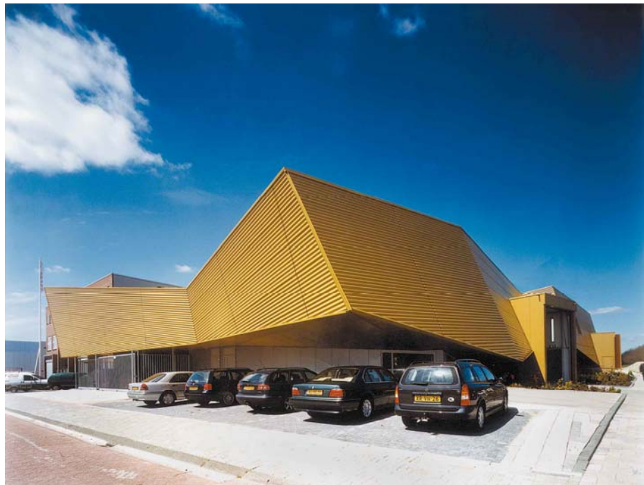
Figure 4.1 Car repair workshop with steel roof and façade
