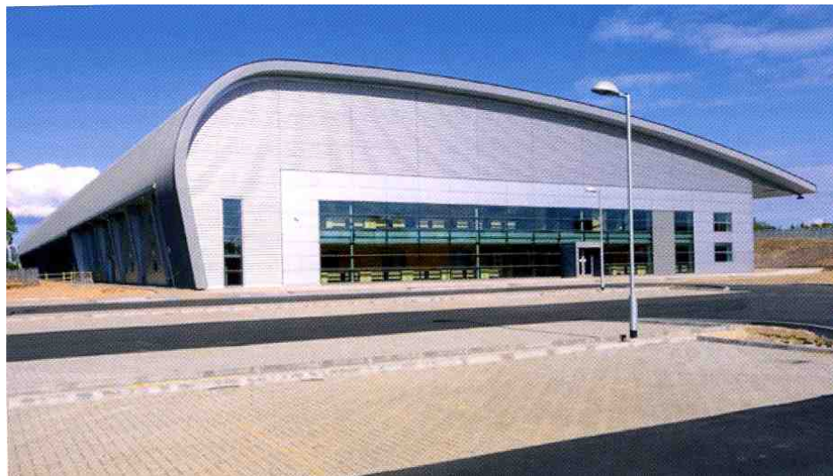
Figure 1.4 Modern industrial building with curved steel roof
