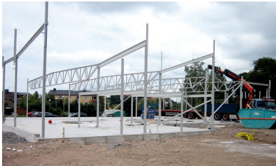
Figure 3.17 Flat truss in pinned frame building
