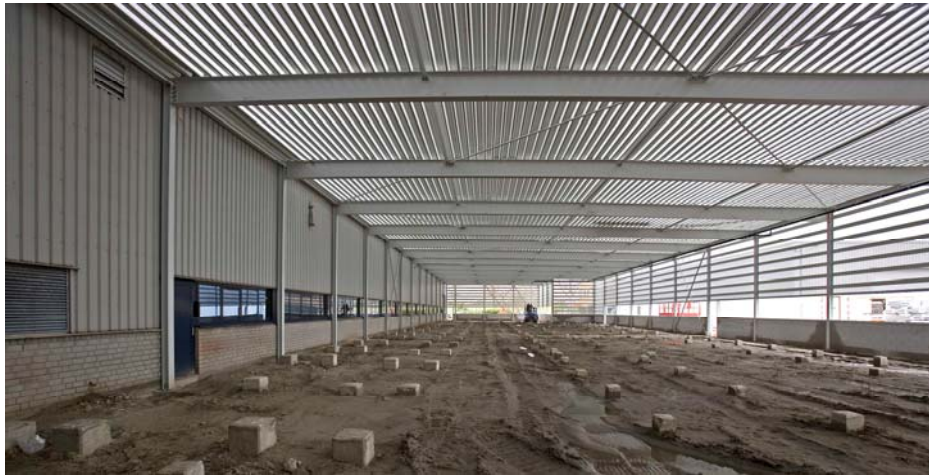
Figure 3.12 Pinned frame beam and column structure
