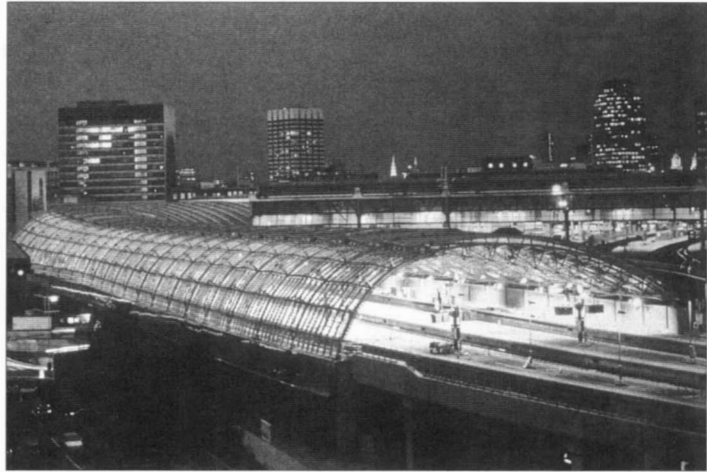
Figure 7.1 General view of Waterloo Terminal
