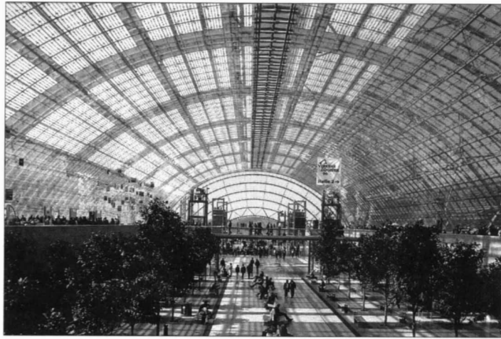
Figure 7.13 Interior view of glass envelope
