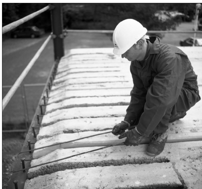
Figure 3.7 U-bars placed around the studs to an edge beam
