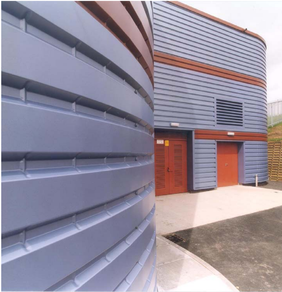
Figure 2.3 Industrial building clad with a combination of horizontal and curved details to produce smooth lines.
