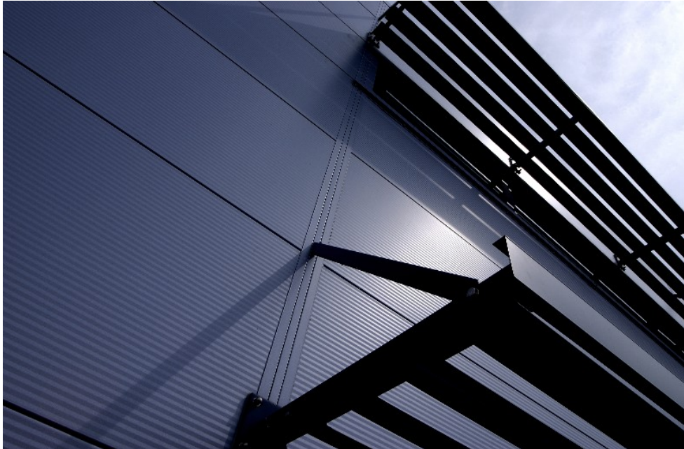
Figure 4.1 An office complex clad with horizontally mounted panels with a micro-rib finish (Photograph by kind permission of Corus P & P)
