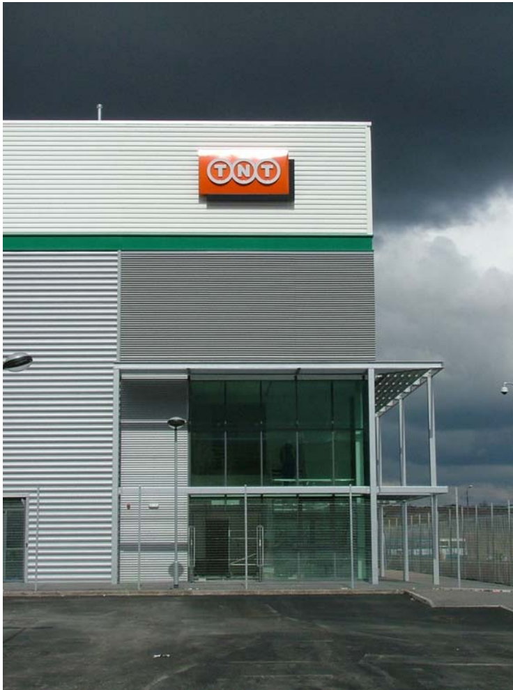
Figure 2.2 The warehouse and office complex has a striking appearance when cladding with different profiles, textures and colours, are combined (Photograph by kind permission of Michael Sparks Associates)
