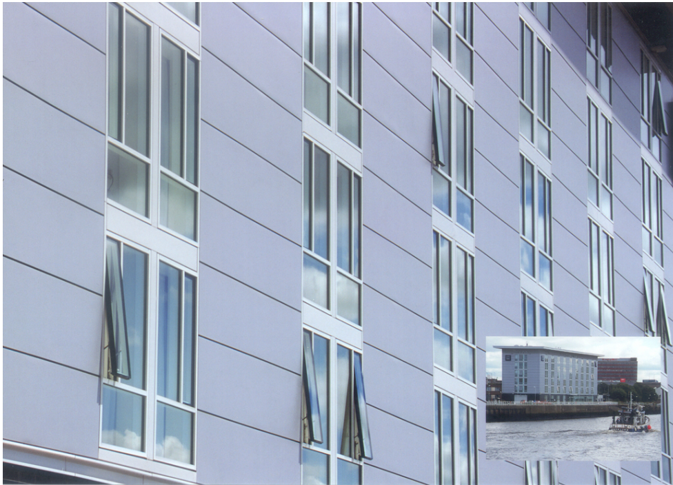
Figure 6.1 Hotel and Inn clad with modular flat panels with fully integrated windows and pre-formed corner panels (Photograph by kind permission of Corus P & P)
