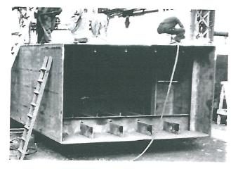
By fabricating the steel units off the site and following a cantilever sequence of erection, congestion on the restricted working area was prevented and the use of land beneath the structures was minimised. The weight of steel in the structure is 12,278 tons of which 10,000 tons is of high yield stress quality.
