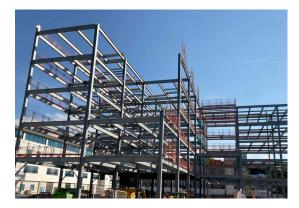
Fabrication and erection required innovative sequencing due to delays in the precast core delivery. Temporary bracing and modified connections allowed the steel frame to be constructed independently, maintaining programme momentum. The long-span stairs were delivered in one piece, requiring precise routing and welding to meet architectural and regulatory standards.
