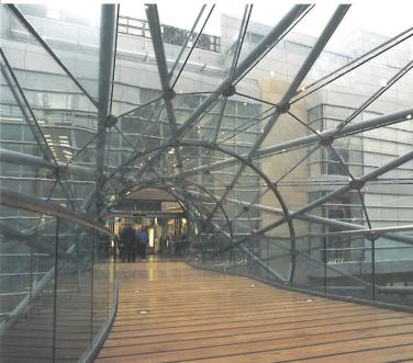
Corporation Street Footbridge has set new standards of structural and façade engineering in urban footbridge design. Innovative techniques range from the use of prestressed steel to form the hyperbolic paraboloid primary structure, to the incorporation of state of the art glazing materials used to ensure public safety in the event of glass panel failure.
