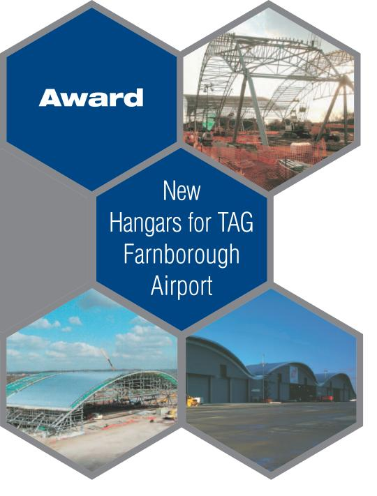
Part of the £45m redevelopment of TAG Farnborough Airport, which also includes a 35m high air traffic control tower and brand new terminal, the £9m three bay hangar is 290m long, 45m deep and 22m high at the apex and large enough to accommodate six Boeing 737s.
