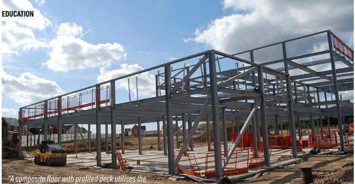
advantages of both steel and concrete. Therefore, it's a more cost-effective form of construction, with a slimmer floor build-up and it's quick to install."
