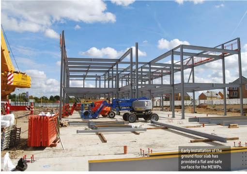
slab was installed, using piles up to a depth of 20m. According to Ingleton Wood Structural Engineer Aakar Saber, this solution was chosen due to the bearing capacity, high shrinkability and dissolution features of the soil, which could have posed a risk of differential settlement if shallow foundations were used.
