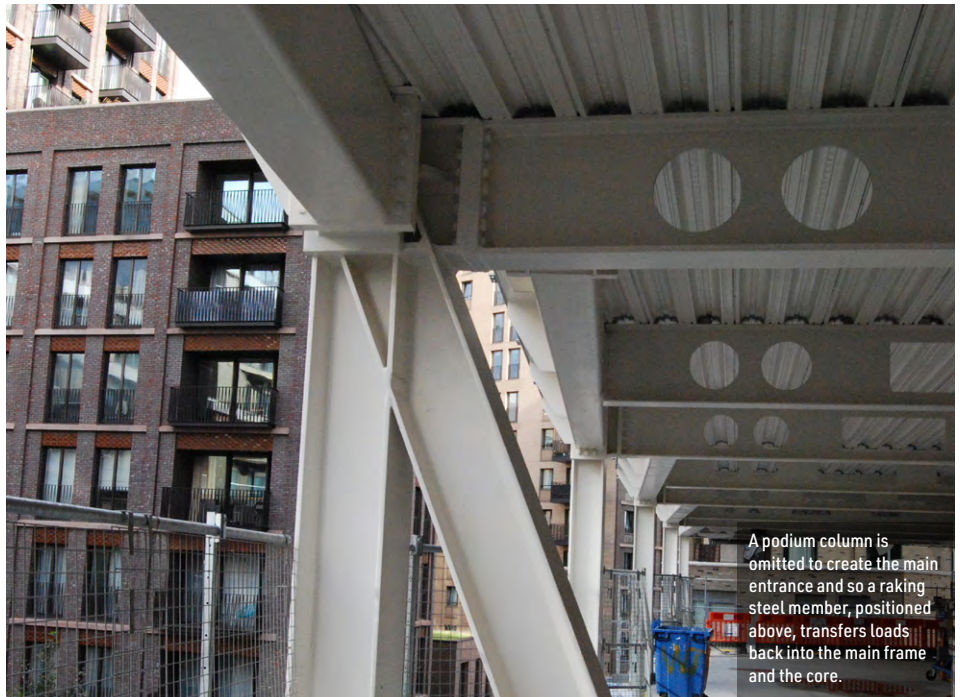
The western office façade features a saw-tooth design, created with offset edge beams that sit between the main columns.
