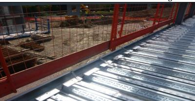
Edge protection installed cantilevered from the beam allows good access for fixing deck edge trim and the shear studs to the top of the beam.
