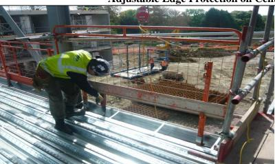
Adjustable edge protection on the centre of the beam with a 460mm gap does allow access to fix the edge trim outside of the beam centre and the shear studs to the top of the beam.
