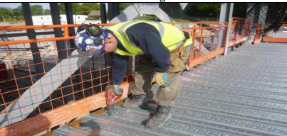
Edge protection on the centre of the beam does not allow access to fix the edge trim outside of the beam centre, or the shear studs to the top of the beam.
