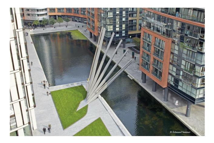
The new moving footbridge at Merchant Square in Paddington is a 3m wide cantilevered structure which spans 20m across the Grand Union Canal, and is divided into five slender 'fingers' which are raised using hydraulic jacks with an action similar to that of a traditional Japanese hand fan.
