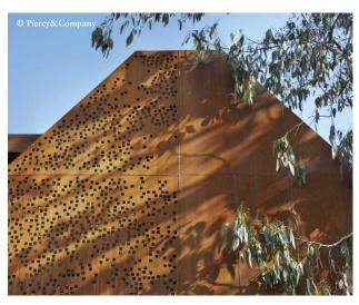
Set within the Kew Green conservation area of south-west London, this four bedroom family house is formed of two prefabricated weathering steel volumes inserted behind a retained 19th Century stable wall.
