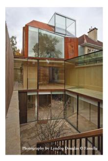
This project involved redevelopment of a garage building in south west London into a high-spec private house set out over four floors including a single basement. The rustlike appearance of the weathering steel cladding is a striking feature of the cuttingedge design of this private dwelling.
