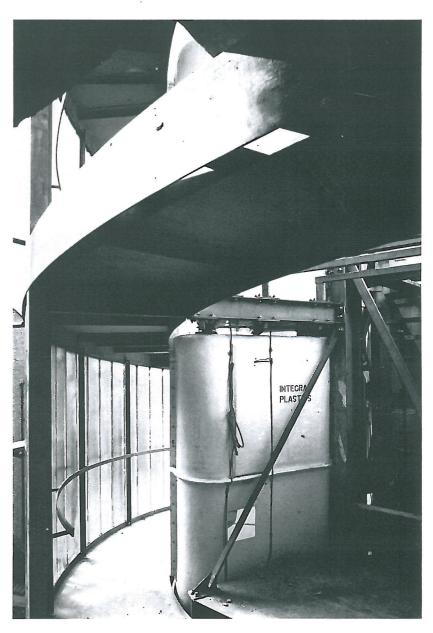
Steel core with some of the glass fibre bathroom units fixed in place.
