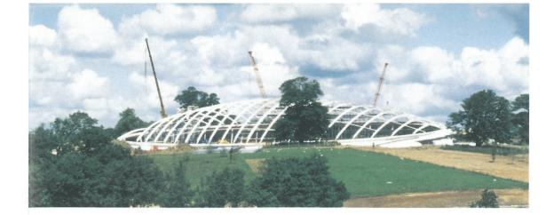
The primary roof member takes the form of a single curved 323 diameter tubular hollow section arch up to 58m long, spanning across the toroid at four metre centres. The arches follow the precise geometry of the toroid, with a constant radius of curvature in every member.
