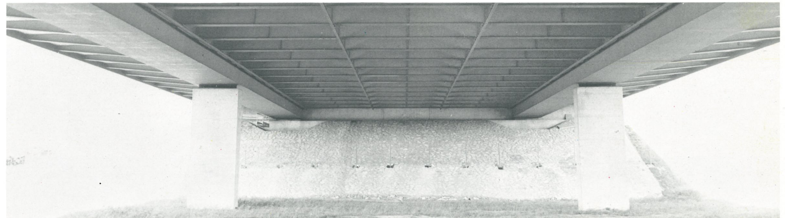
Below: The bridge structure showing transverse beams and continuous box-girders.
