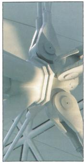
which rise up through the floor - the 'trunks' of the structural trees.
