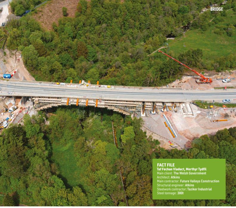
The steelwork package has been divided into three phases, with each one installing six complete beams. The initial phase involved the centre of the viaduct.
