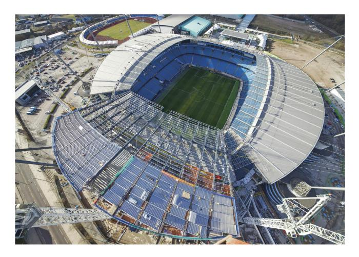
The South Stand expansion increased the capacity of the stadium during the 2014/15 football season, adding 6,000 new seats through a third tier on the terraces and 1,500 additional seats around the pitch. An architecturally sympathetic extension of an existing catenary ringed structure was needed, which did not compromise the integrity or capacity of the structure and ensured that the existing stadium remained operational during works.
