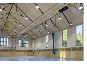
Height restrictions for the sports hall roof, from both above and below, led to a creative double-pitched solution with no central support using four sloped steel trusses which span 34m along the length of the building.
