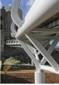
the possibility of weld distortion in the fin plate attached to the CHS. An alternative solution was adopted whereby SHS bracing was used and the handrail fabricated tee upright orientation was reversed. The face of the SHS Vierendeel bracing then aligned with the flange of the tee to the balustrade which was tapered to give an elegant transition to the handrail, whilst the bracing also gives improved structural capacity particularly at the joint with the CHS chords for a given section width.
