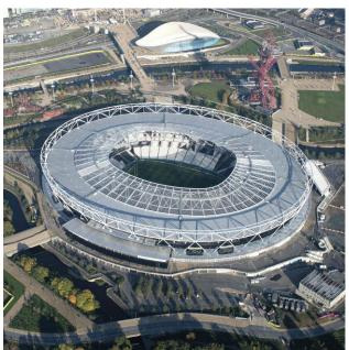
Strengthening of the existing structure was one of the major challenges. Due to the additional weight of the new roof, it was necessary to replace and/or strengthen the existing V-columns and significant strengthening works were carried out to the existing compression truss.
