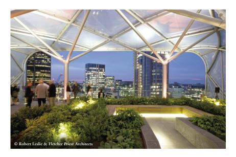
The striking roof canopy provides allweather protection for the 204m<sup>2</sup> sky court. The tubular steel and fritted ETFE canopy frames views out in two directions over central London, wraps up and over the garden and extends four storeys down the face of the southwest façade in a diagrid to assist solar shading.
