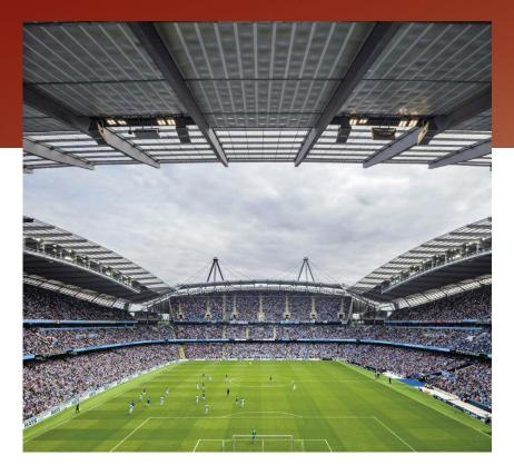
The project contains a number of highly bespoke details tuned to the complex geometries and design challenges, including the multi-stay connection at the top of the masts and column bases formed of spherically machined plates and rotational bearings, which allow the new design to accommodate differential movements between the new and existing structures.
