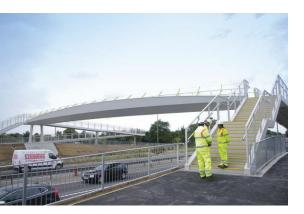
The structure is a steel hybrid box girder/halfthrough trough. This efficient structural form gives both excellent torsional rigidity and allows the bridge to have a low overall structural depth.
