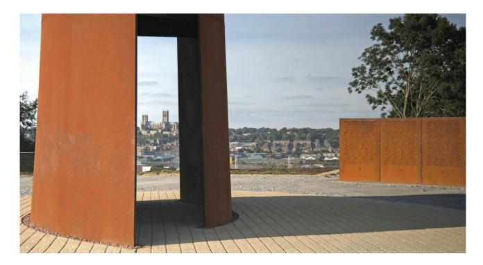
Steel was the obvious choice for the Spire and the weathering steel plate fulfilled all the structural and aesthetic requirements of the project. The selection of weathering steel gives the Spire a cold austere feel which, whilst not requiring applied surface treatments, will be maintenance-free throughout its lifespan.
