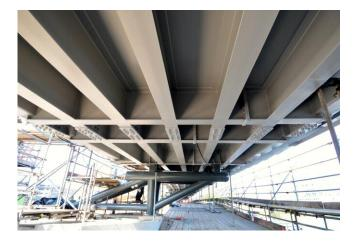
gates which control the flow of the water in and out of the river Lagan. These 'Pier Houses' were to become the main support points for the new footbridge. The bridge is connected to them via four steel truss-type frames or 'trees' made from CHS sections, each of which was unique as a result of the bridge being curved in two directions.
