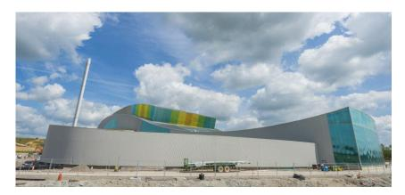
The facility has been constructed to treat 300,000 tonnes of non-recyclable waste each year, diverting at least 95% of Oxfordshire's residual municipal waste away from landfill and generating enough electricity to power 38,000 homes.
