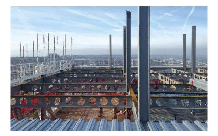
Located in the heart of Reading town centre, the existing Thames Tower concrete office block has been given a new lease of life with an enlarged footprint at each floor level in conjunction with a five-storey steelframed extension above level 11.
