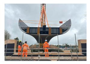
clearance below, semi-integral bearings, and a durable exposed aggregate road surface edged in Blue Lias stone. The steelwork was fabricated in 12 transportable sections, reassembled on site and then lifted into place using a 600 tonne crane, with site safety and logistics expertly managed throughout.
