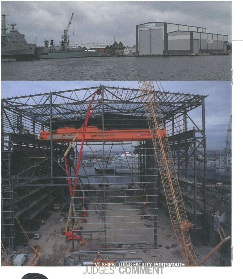
An important maritime manufacturing facility located in this historic naval dockyard. This is an industrial building on an impressive scale, housing two tiers of heavy-duty overhead cranes. It is the marriage of traditional steel structural forms, scaled-up to optimise the use of secondary framing components that has produced this most efficient structural design solution.
