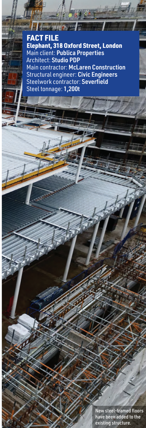
Some of the original columns have been reused in the scheme.
