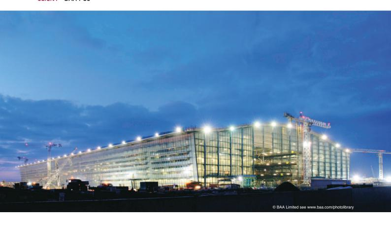
BAA commissioned a new terminal, T5, to handle an additional 30M passengers per annum. The design was a direct reaction to BAA's desire to create a building that would be an aviation landmark and could adapt over time to the ever-changing requirements of the industry. The single span provides a coherent building envelope while remaining independent of the building's internal superstructure.
