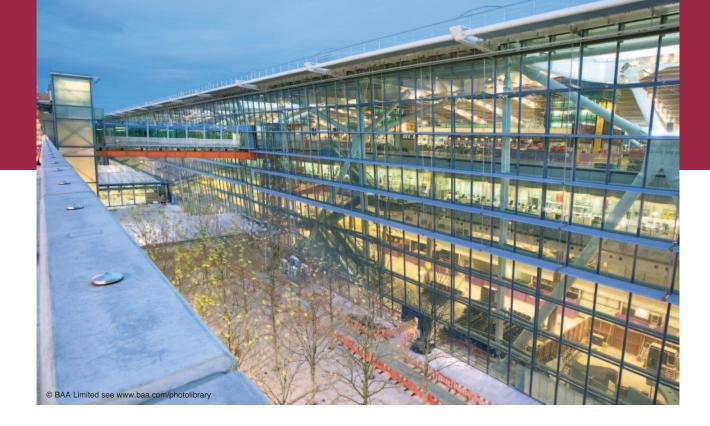
rafter ends complete the 3D hybrid portal frame structure. The splices in the central arched section of the rafters always carry net compression. Therefore, they can transfer forces from section to section in bearing. No welding is required. 120mm diameter "male" and "female" shear connectors interconnect during erection so that the whole rafter fits together like giant Lego bricks. As a result the splice is almost completely invisible but is very quick and easy to build.
