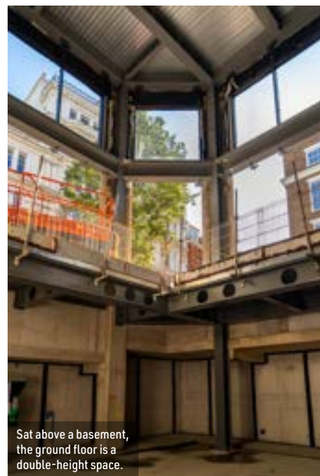
Creating an efficient floor design, building services are accommodated within the beams.
